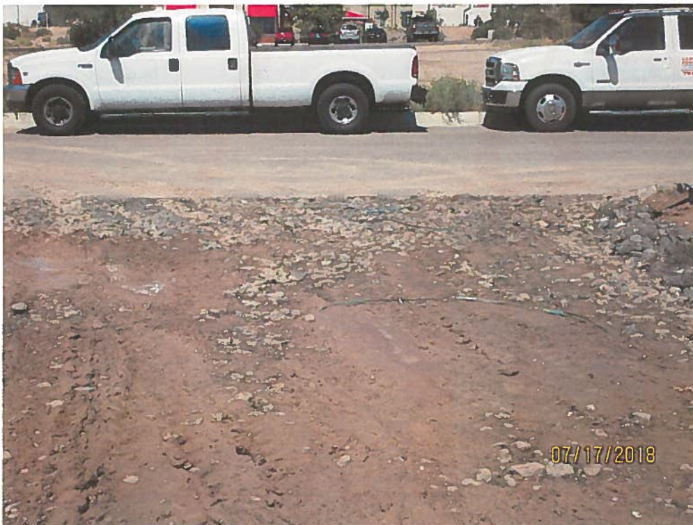
Track-out pad requires maintenance/replacement.
