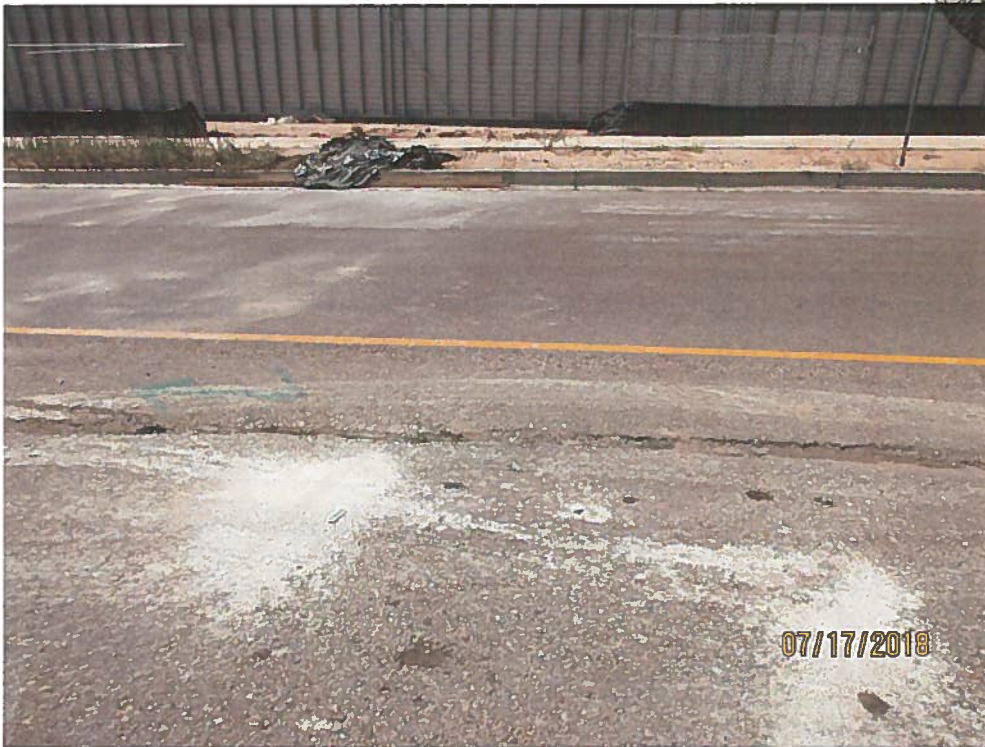
Cement material on La Orilla Rd. Silt fence was removed for access.
