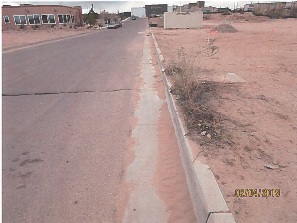
Sediment in gutter.
