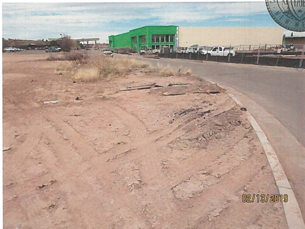
No silt fence east edge of site.
