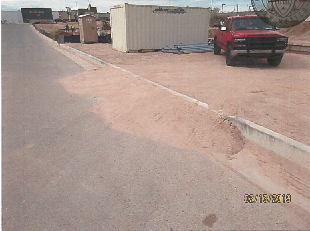
Dirt ramp in street and no vehicle tracking control.
