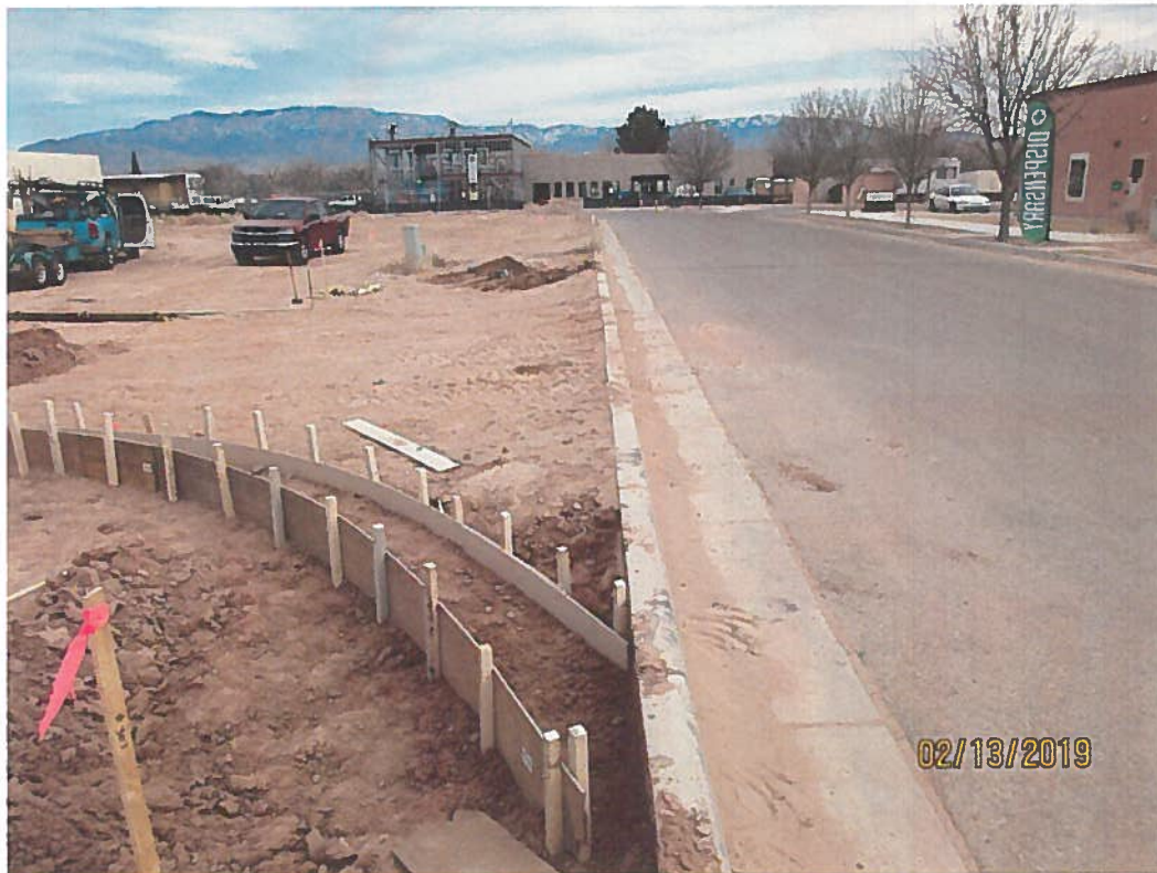
No silt fence south edge of site.
