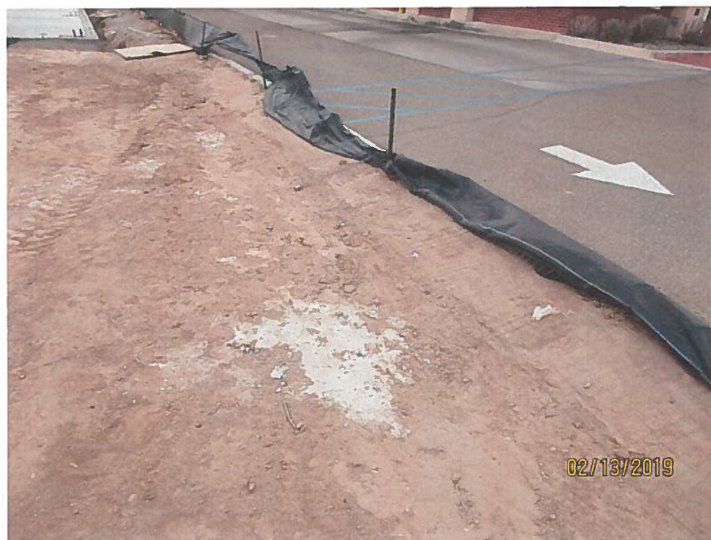
No silt fence east edge of site.
