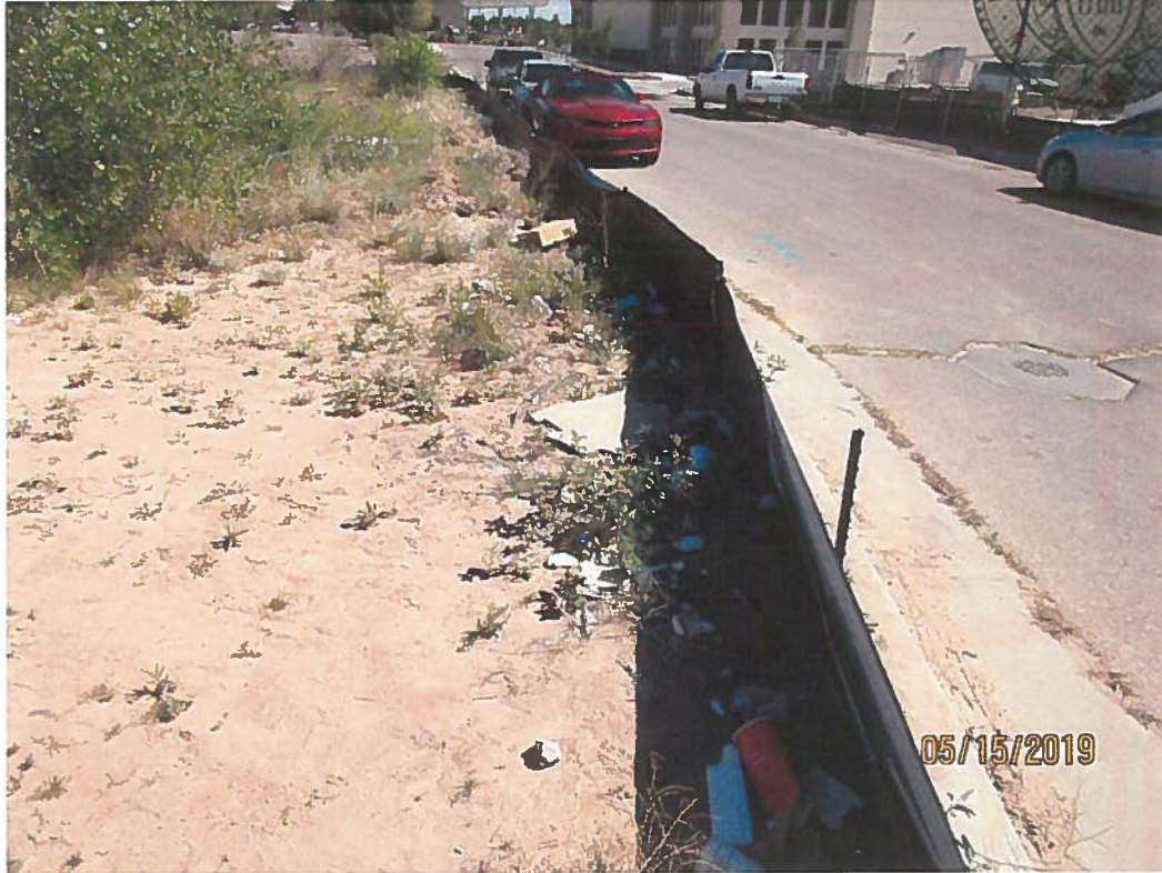
The silt fence along the east edge of adjoining property is a continuous area of waste.
