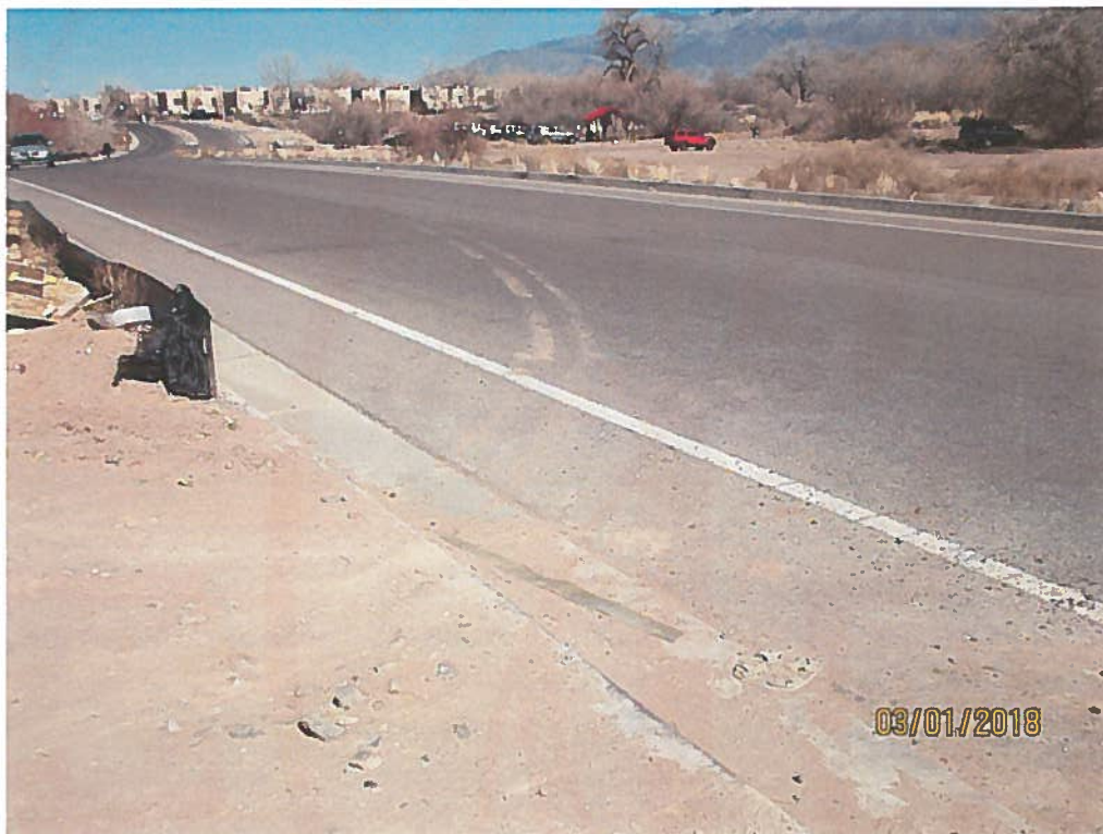
Track-out onto Mirandela St.
