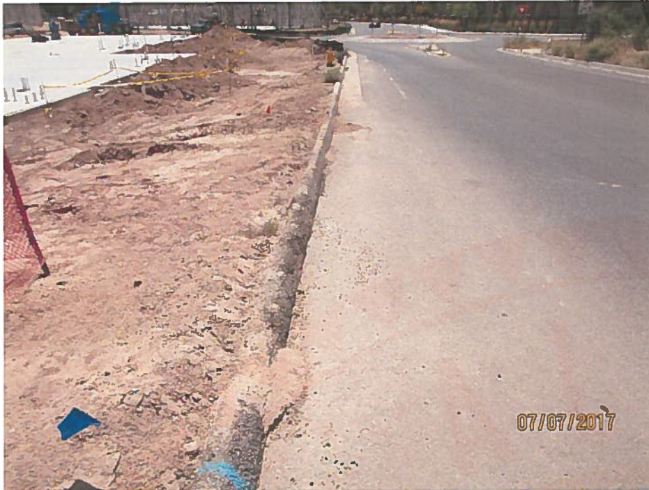
No sediment BMP and sediment spilling into street.
