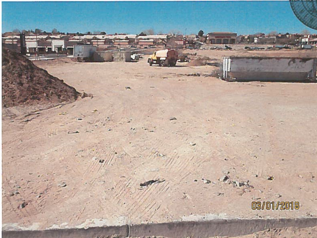
Different view of no track-out pad from staging area.
