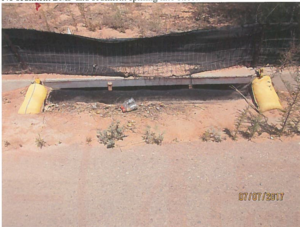
Inlet protection requires maintenance.
