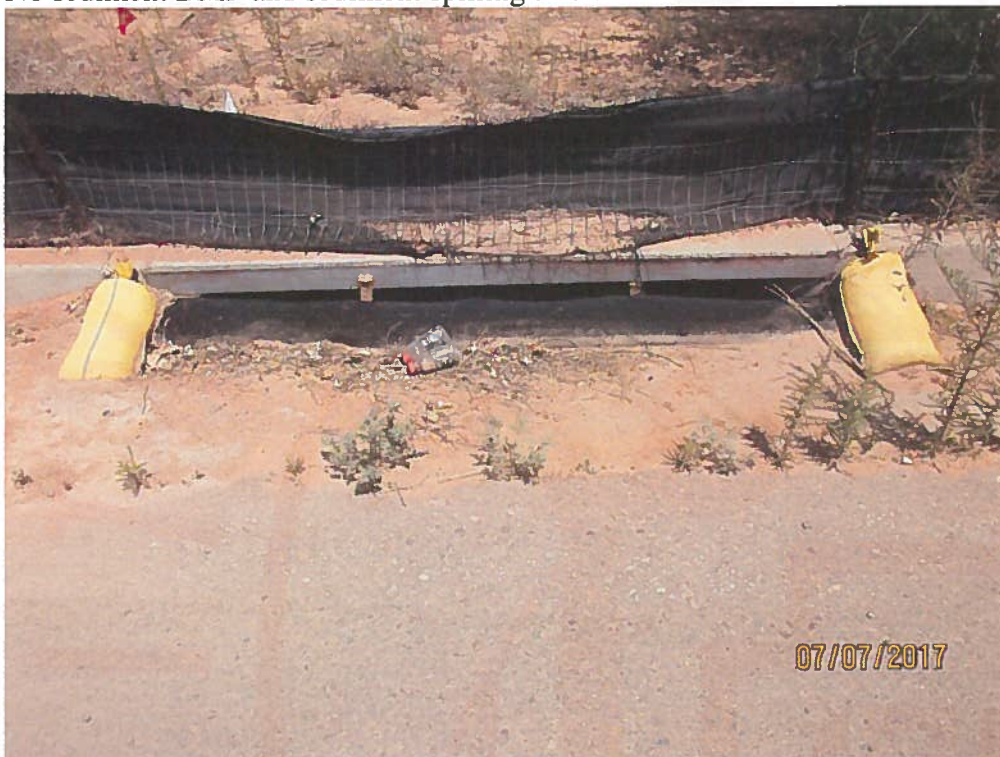
Inlet protection requires maintenance.
