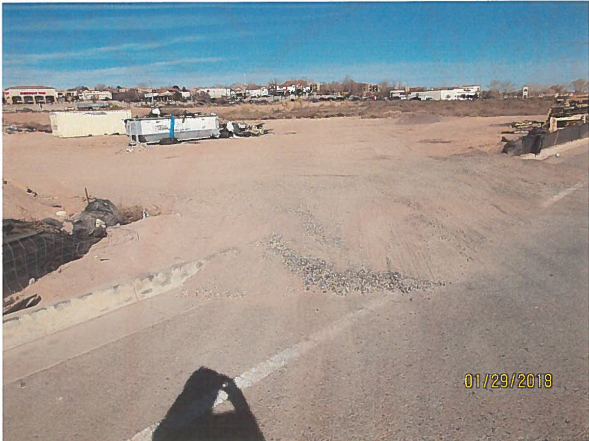
Dirt ramp in street and no track-out pad.
