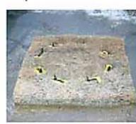
3. Position the mat. Place Inlet Filter on grate with the net side down, flush to the back edge and extending beyond the grate opening on the front and both sides. The zip ties attach Inlet Filter to the inlet grate cover WITHOUT LIFTING THE GRATE COVER.
