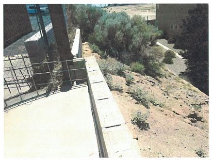
If leaves and debris accumulate on the chain link fence on Lot 4 of the **SEGO-COX Subdivision** it could back water up on the leaking wall and increase the leakage. The drainage swales in the SEGO-COX Subdivision should not be blocked by leaves and debris. Redesign and/or relocation of the fence is recommended. Maintenance is the responsibility of the current owner of record,
