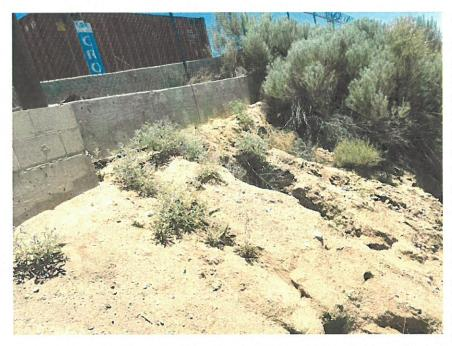
The footing of the wall does not appear to be deep enough to prevent leaks. Furthermore drainage can easily infiltrate through the dirt gap between the wall on Tract J-1-A and the asphalt paving Lot 4 of the Sego-Cox Subdivision.
