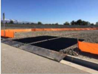
SEDIMENT TRACK OUT CONTROL
