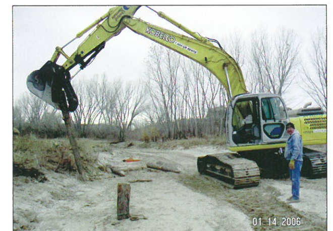
Photo 5-14. Excavator with a "thumb" used to push log vanes into riverbed. Rio Puerco, Sandoval County, N.M. (Photo by Mike Chavez)
