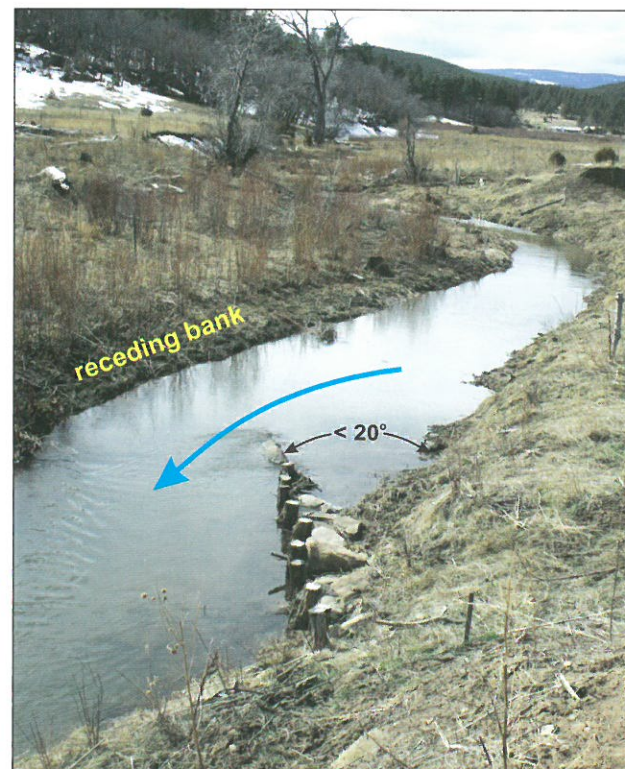
Photo 5-10. A post vane, manually installed, on perennial Manuelitas Creek, San Miguel County, N.M. Note that the opposite bank is beginning to recede. (Photo by Tamara Gadzia)
