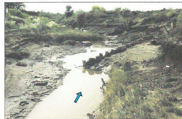
Photo 5-9. The first ever post vane, 1999, used to initiate erosion of the opposite bank, Pueblo Colorado Wash, Apache County, Ariz. Note deposition upstream and downstream from the vane, downstream deposition not visible. (Photo by Bill Zeedyk)
