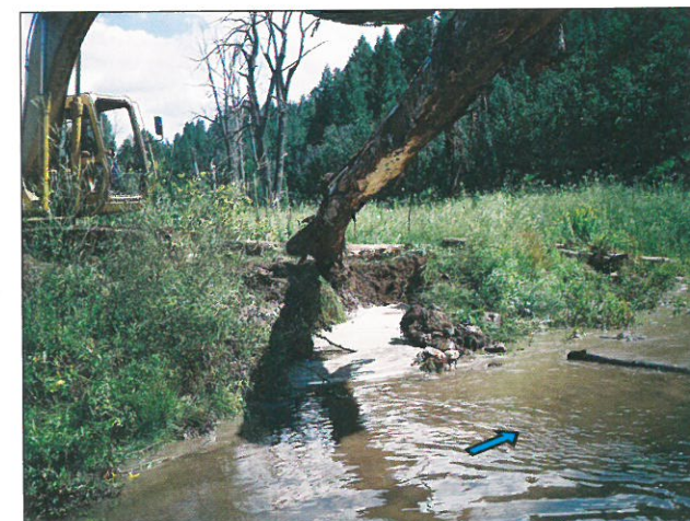
Photo 5-19. Using an excavator to install a log vane on Manuelitas Creek, San Miguel County, N.M., August 2005.
