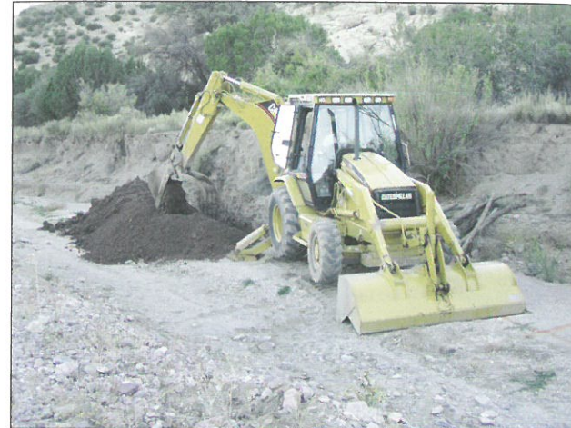
Photo 5-16. Installing a post vane in an ephemeral channel using a backhoe to dig a trench while the stream is dry.
