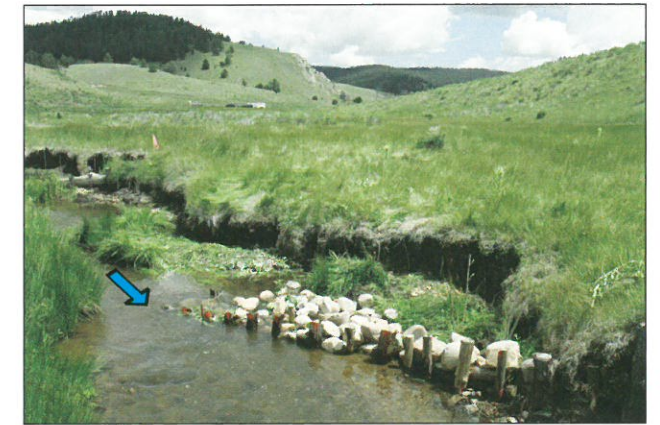
Photo 5-12. The vane/bank intersection is filled with rock and sedge wads to initiate the formation of a bankfull bench. Comanche Creek, Taos County, N.M. (Photo by Courtney White)
