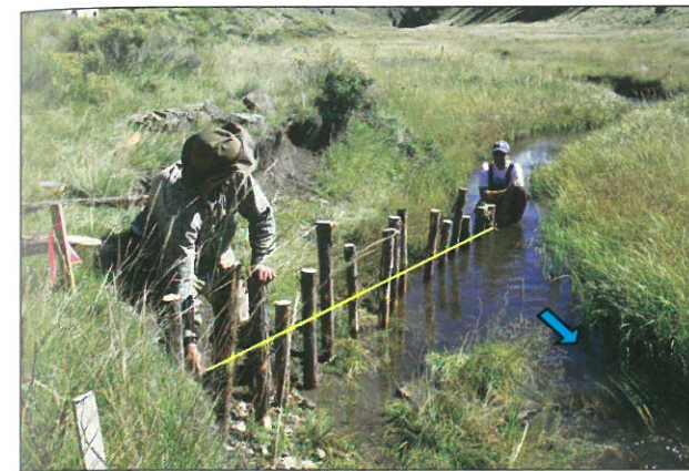
Photo 5-11. Stretching a string to mark the line of descent on a post vane. Comanche Creek, Carson National Forest, Taos County, N.M. (Photo by Tamara Gadzia)
