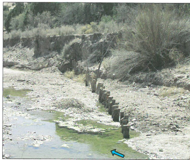
Photo 5-18. Installed post vane. Stream is flowing after first flood. (Above photos by Van Clothier)
