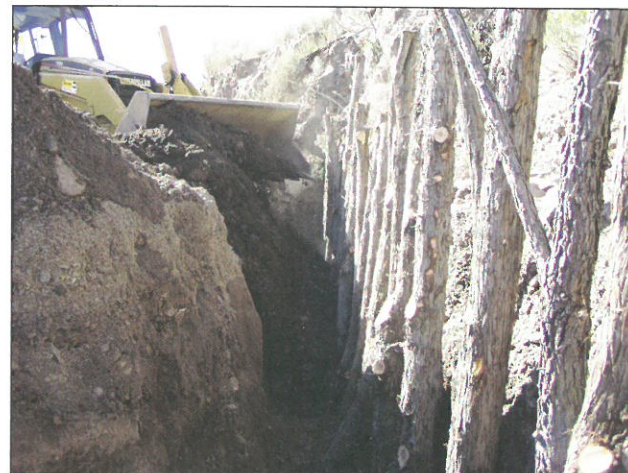
Photo 5-17. Placing excavated material in the trench alongside the posts. Note: this sequence shows posts on bank side of trench. Placing them on the stream side of the trench is more secure.
