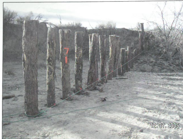
Photo 5-15. Mechanically installed posts scribed at the proper angle for trimming. Rio Puerco, Sandoval County, N.M. (Photo by Mike Chavez)
