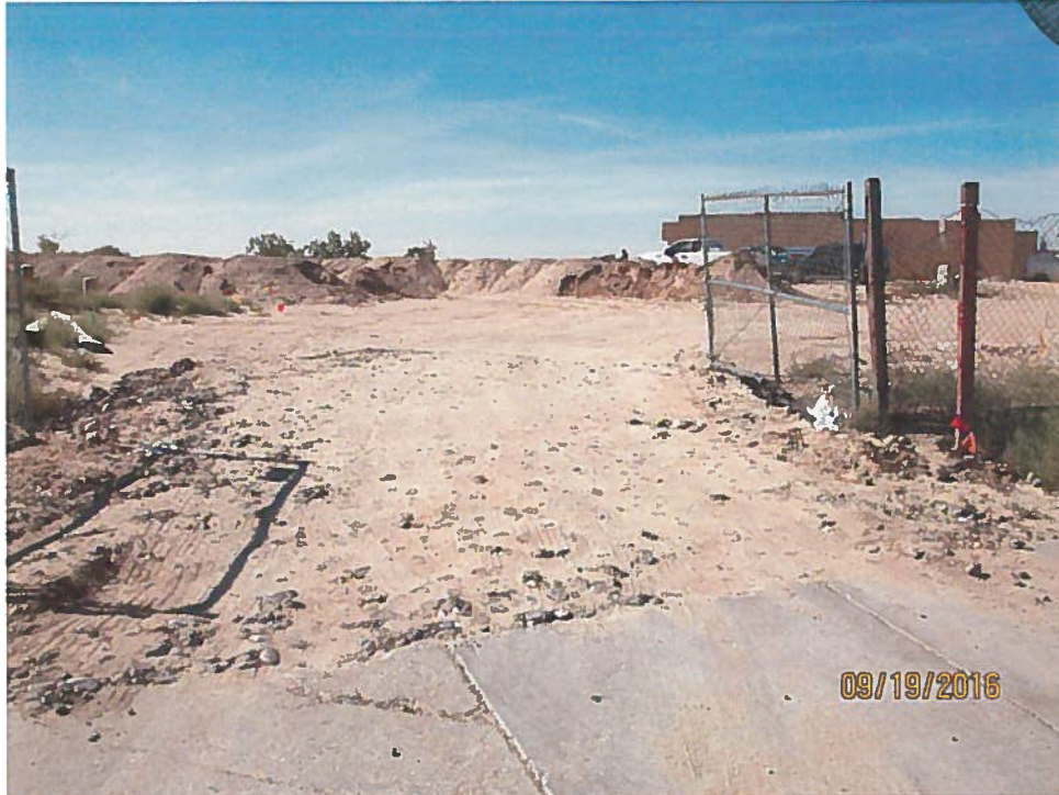
Construction entrance to the site poorly maintained.
