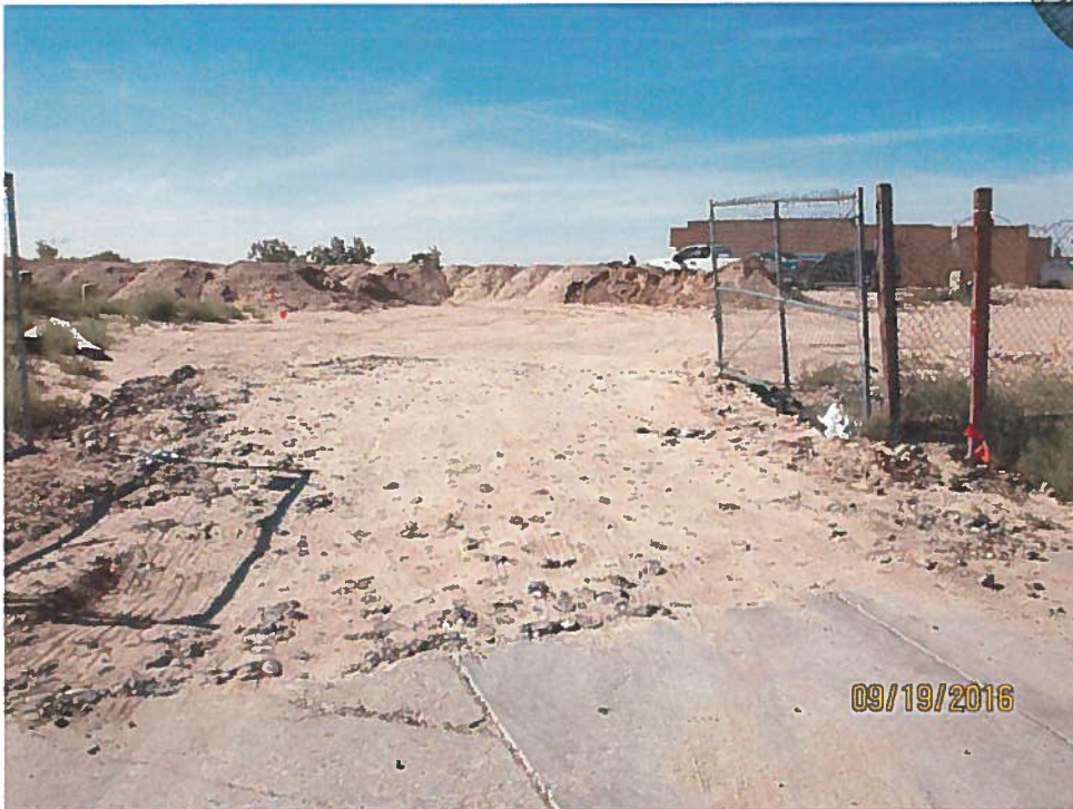
Construction entrance to the site poorly maintained.
