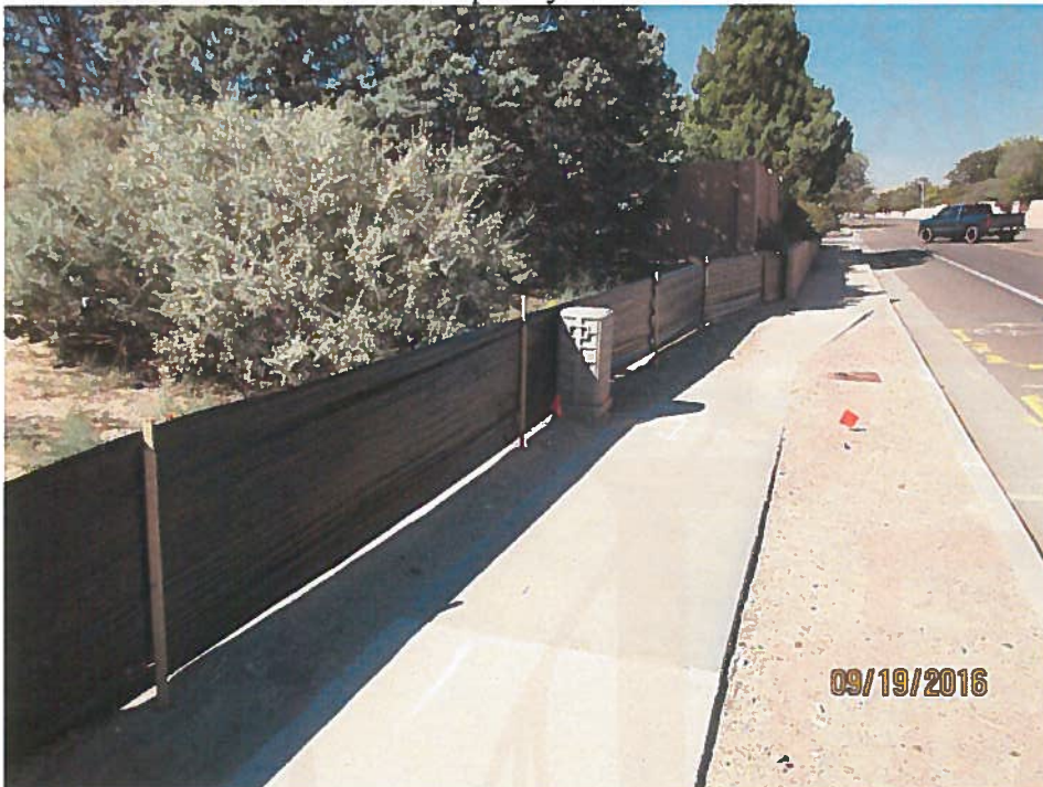
Silt fence along Dellyne Ave. not buried; ineffective.
