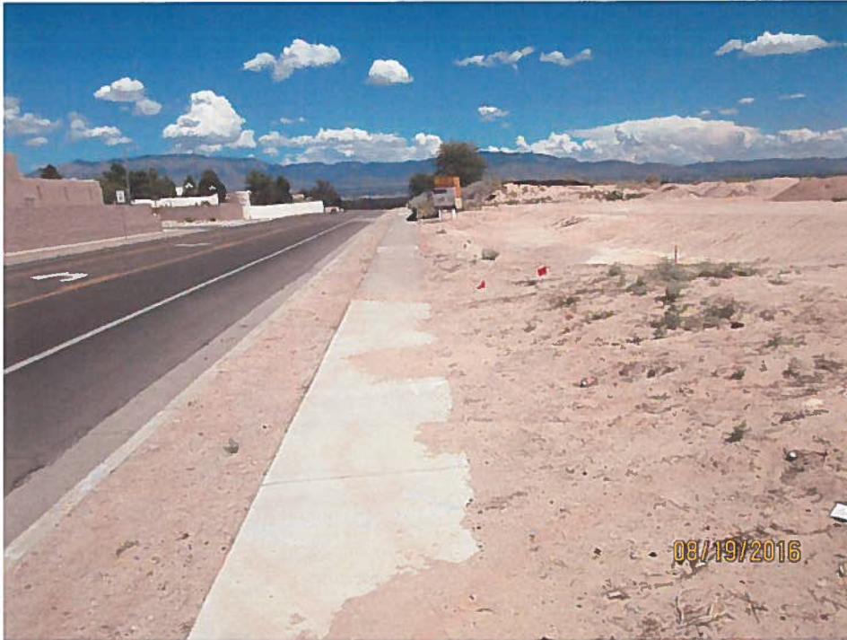
No silt fence along Dellyne Ave. Sediment leaving site.
