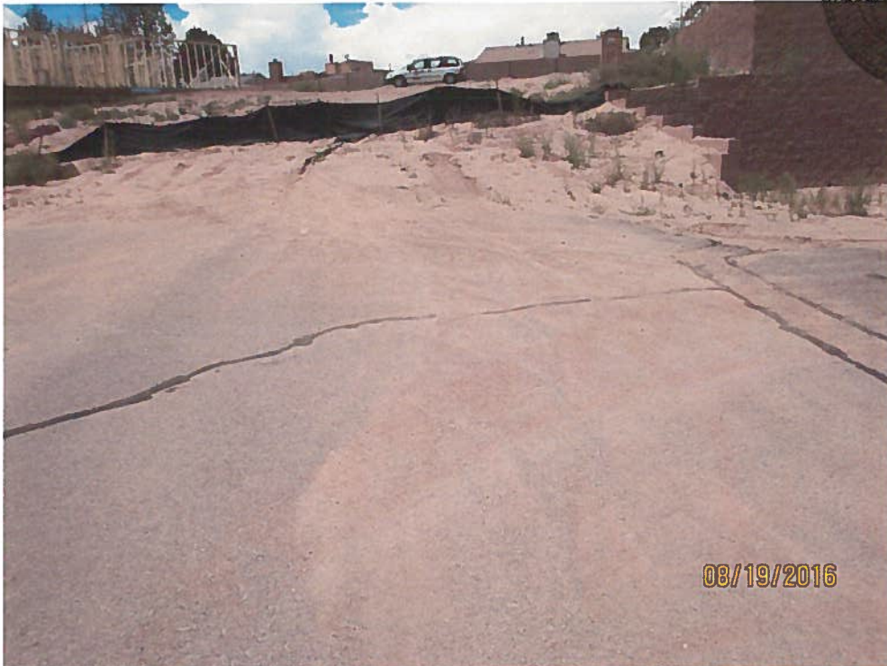
Sediment in Mill Rd. from ineffective BMP not per approved plan.
