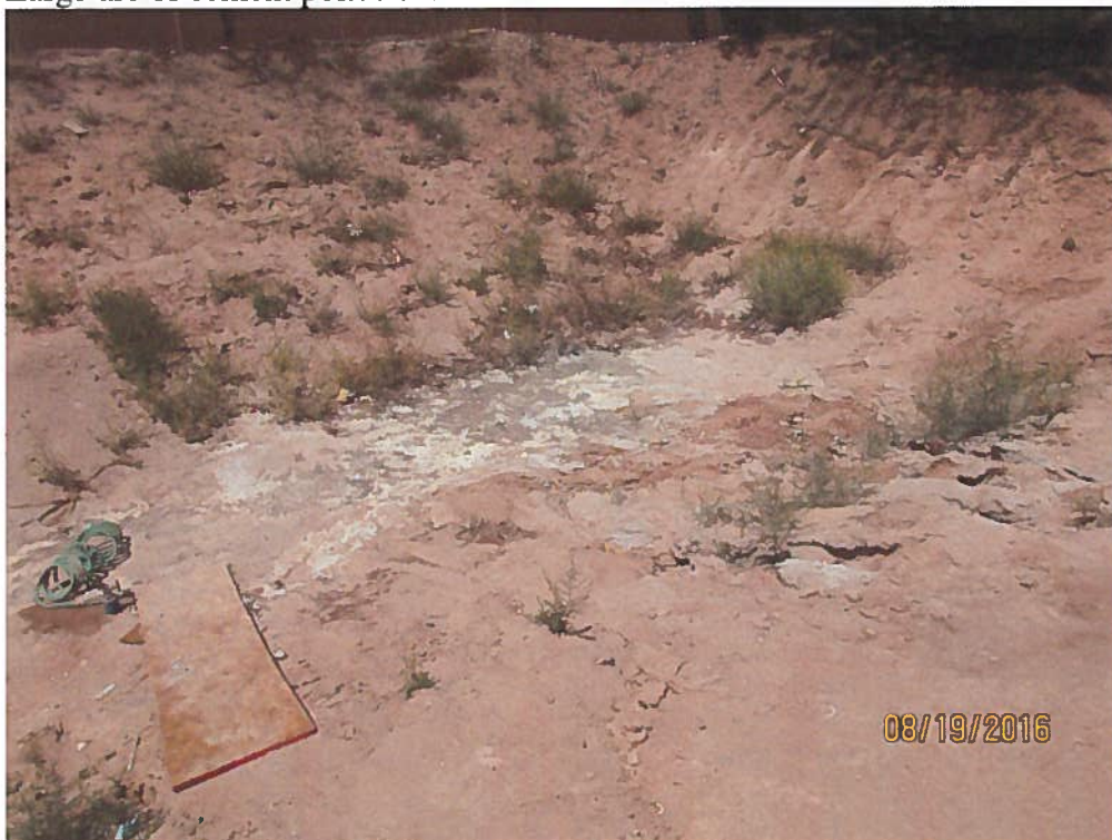
Cement pollution in ponding area.
