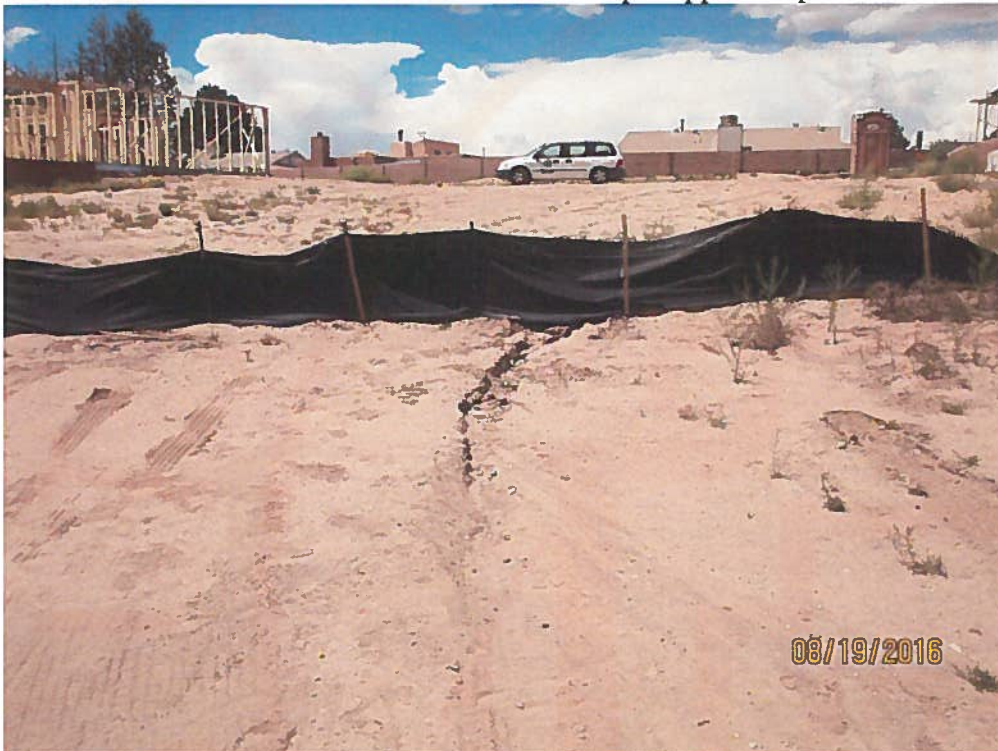
Erosion from ineffective BMP not per plan.
