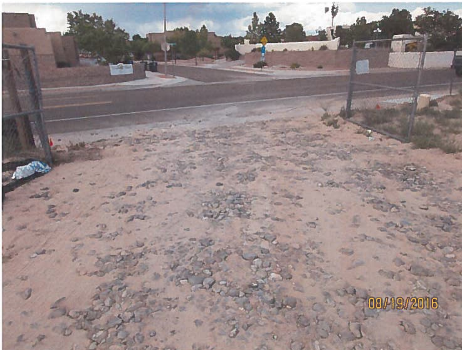
Construction entrance not maintained.
