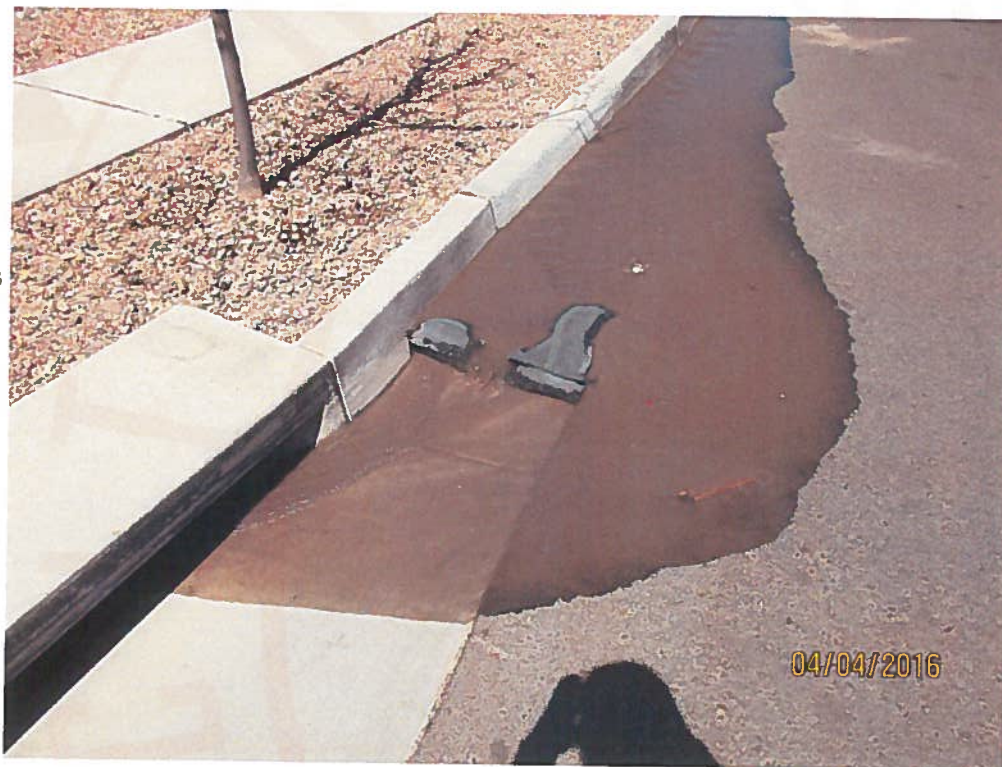
Rinse water flowing into inlet in Calle Espana NW. Inlet protection not filtering water.
