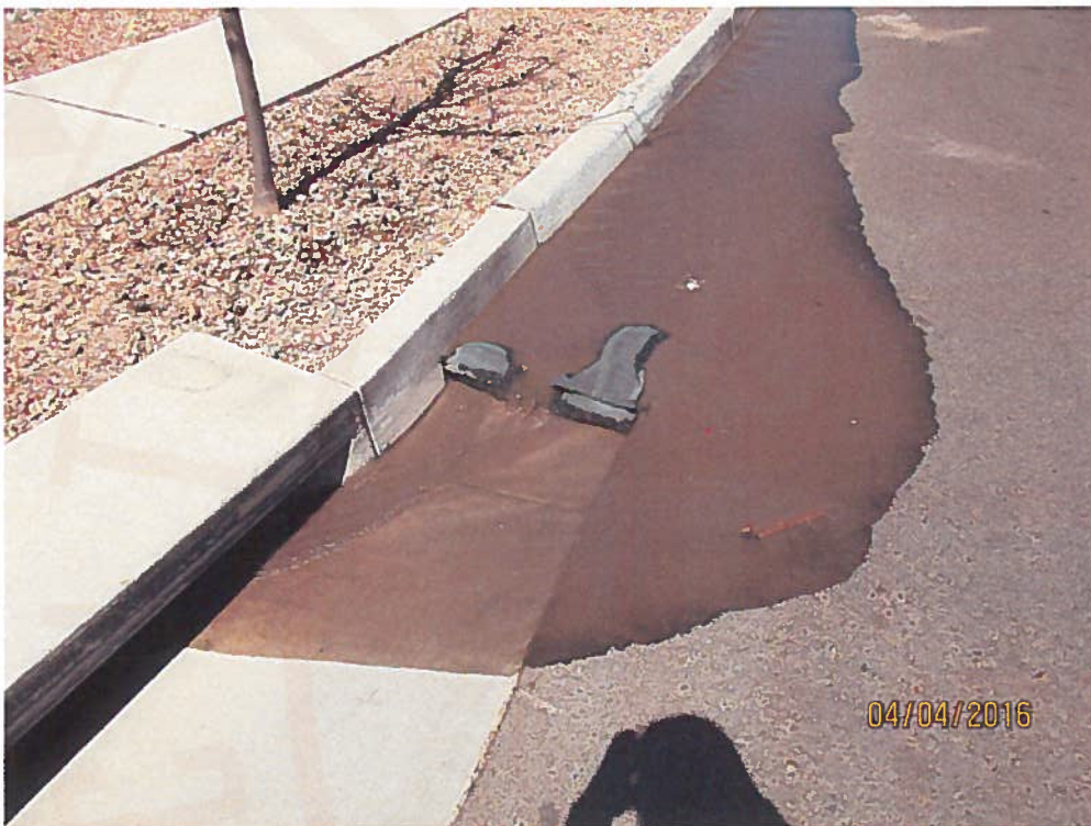
Rinse water flowing into inlet in Calle Espana NW. Inlet protection not filtering water.
