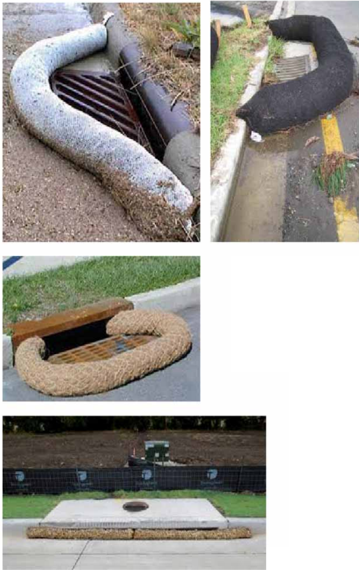
Curb Storm Inlet Protection with Wattles
