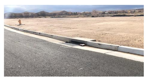
Provide inlet protection for curb inlets on internal roadway.
