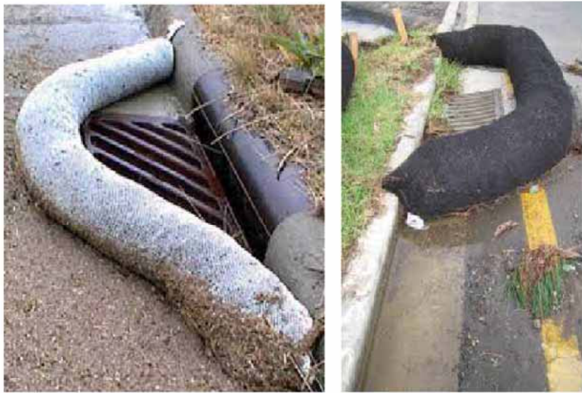
Curb Storm Inlet Protection with Wattles
