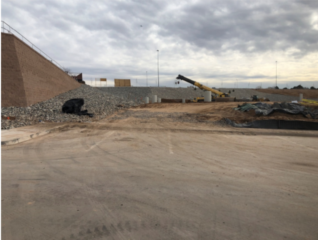
Re-establish Rock Exit
