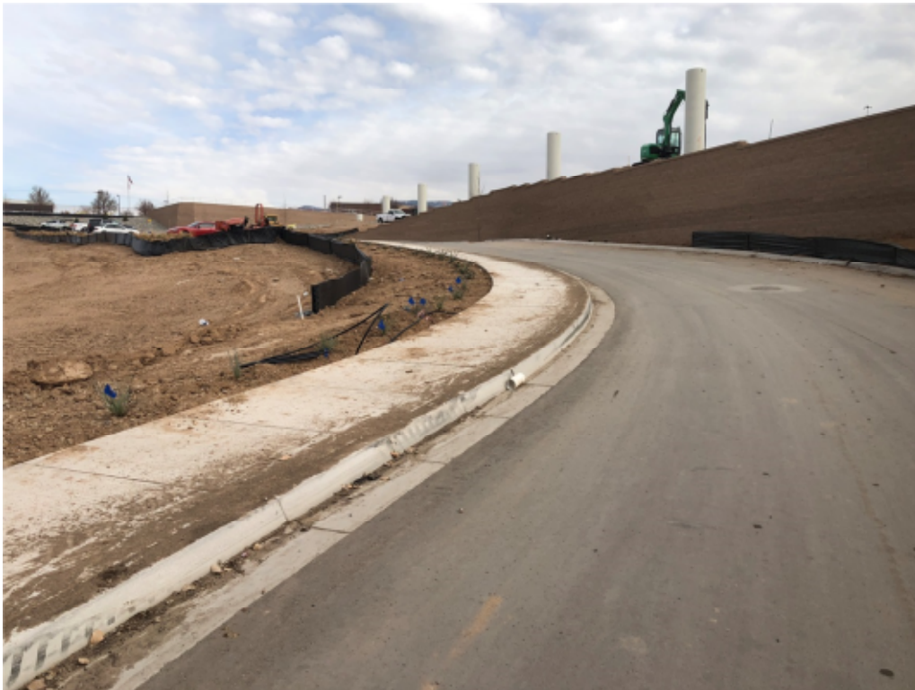
Sweep Clean Sidewalk and Roadway
