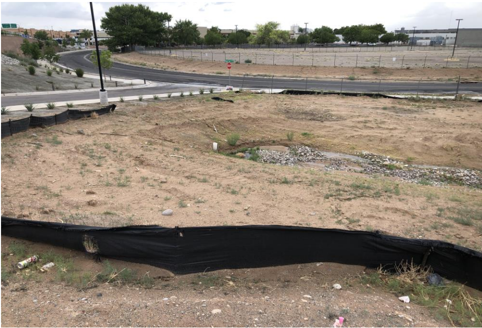
Silt Fence repairs needed
