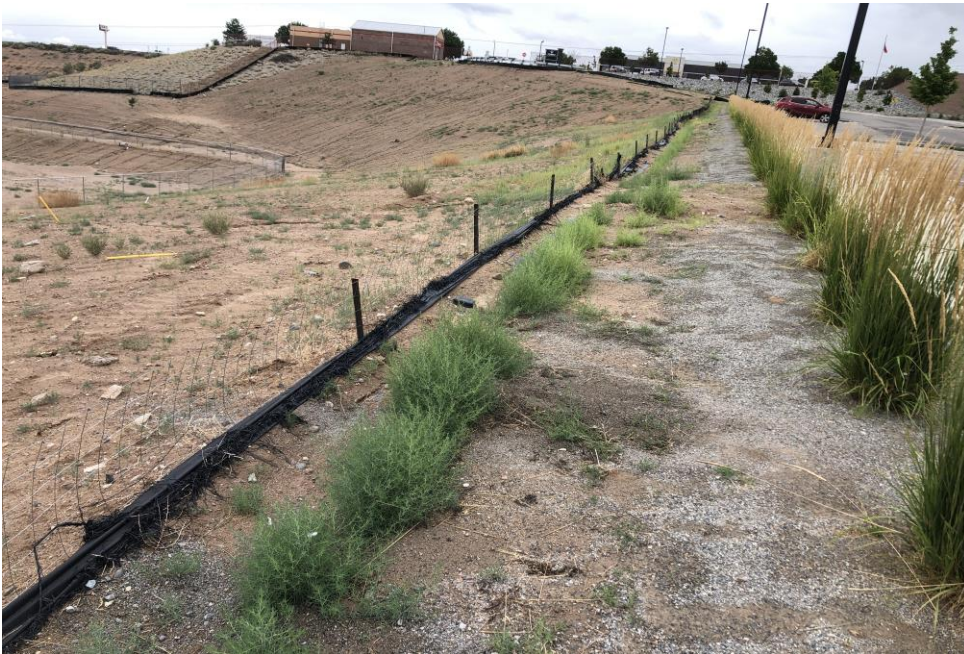
Silt Fence repairs needed
