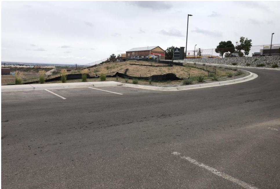
Silt Fence repairs needed
