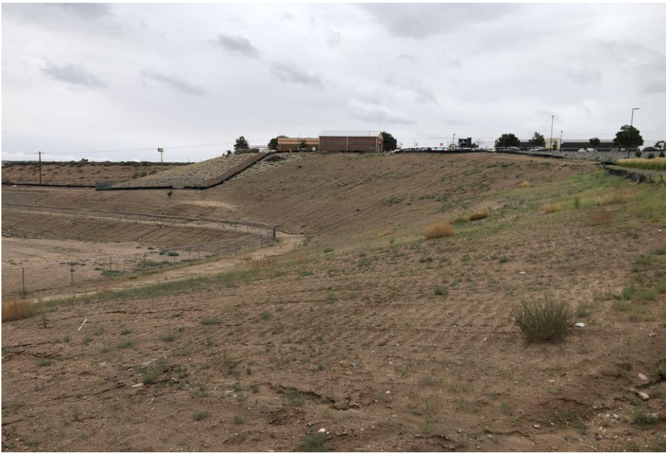
Slope Stabilization Required
