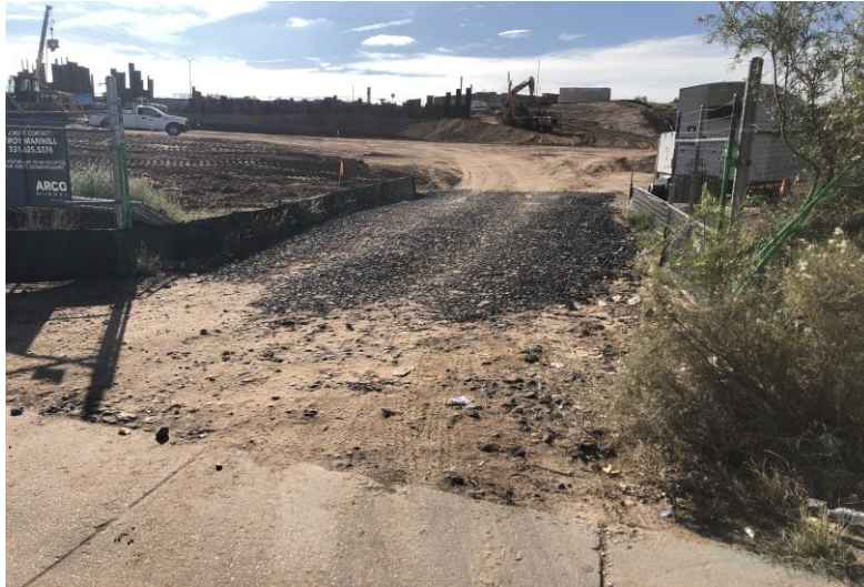
North exit requires larger rock to control sediment track out
