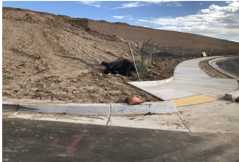
Replace Silt Fencing
