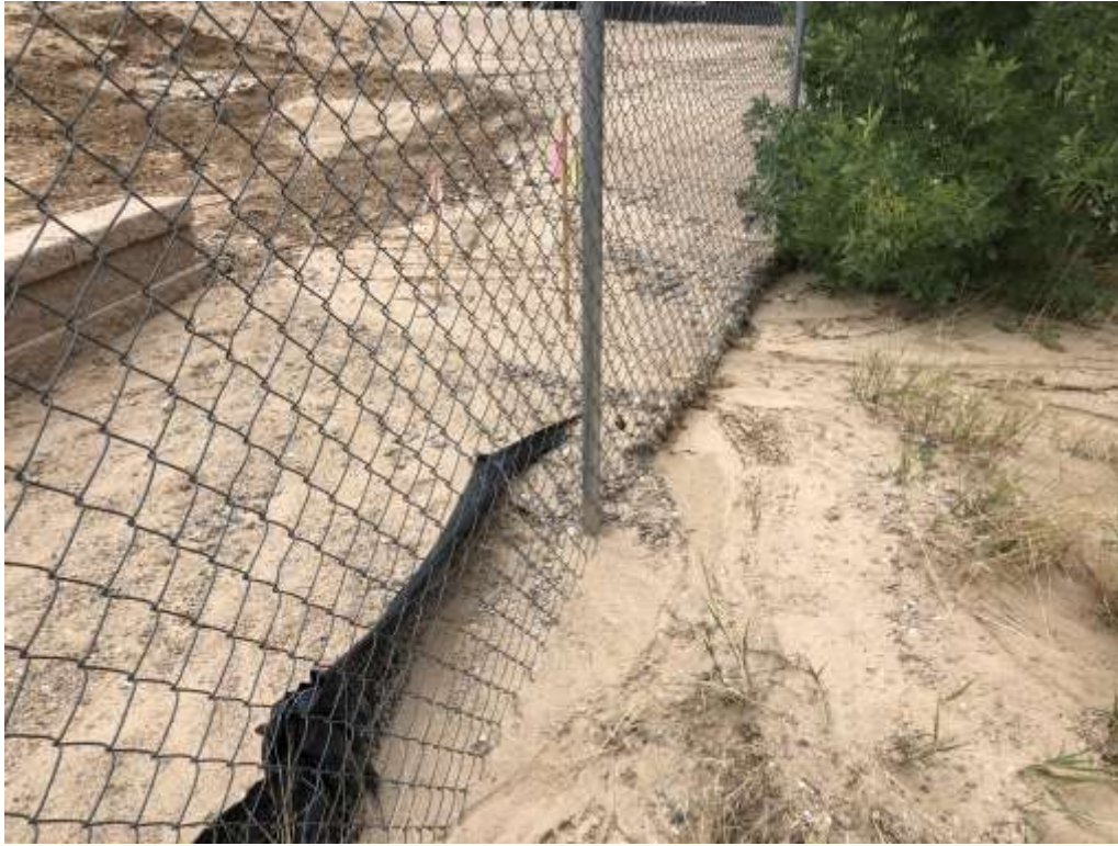
Silt fencing over capacity
