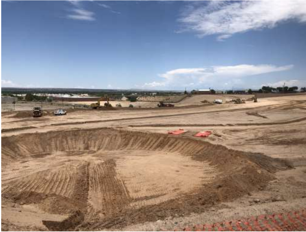
Run-on receiving pond requires dedicated emergency overflow
