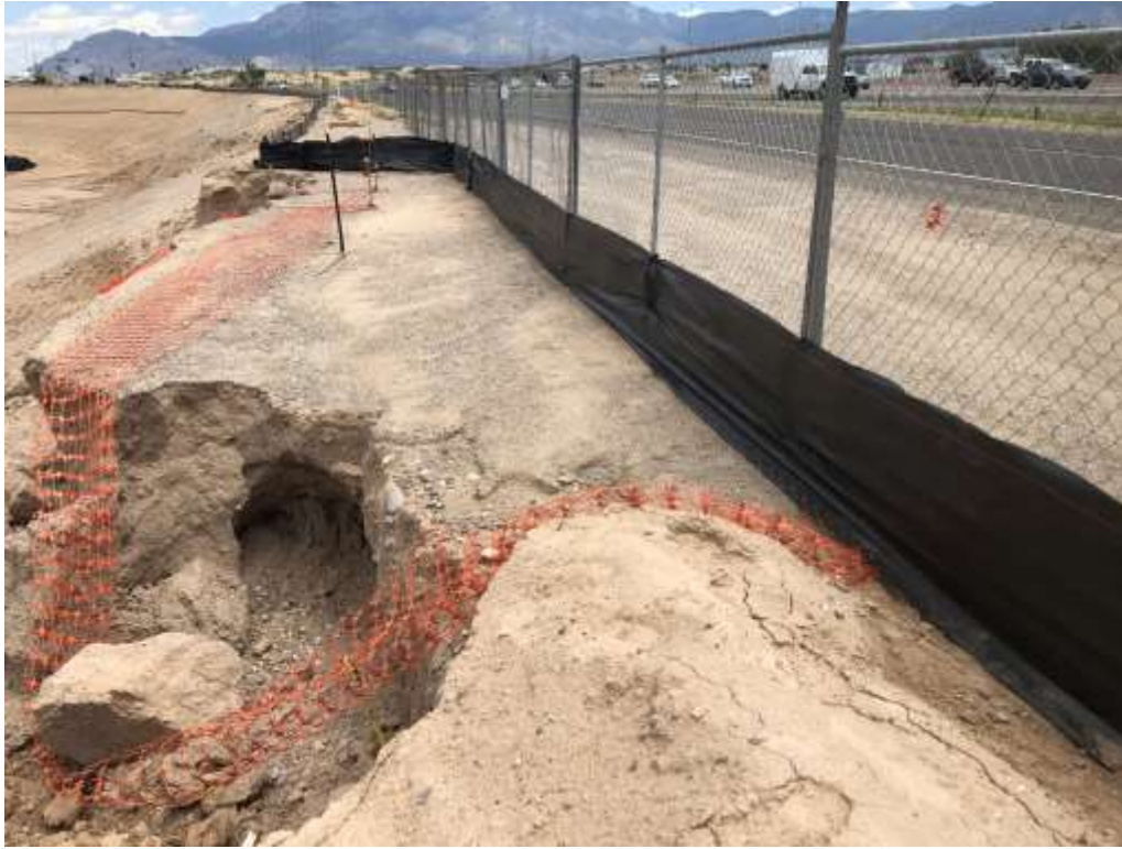
New silt fencing not keyed into sub-grade
