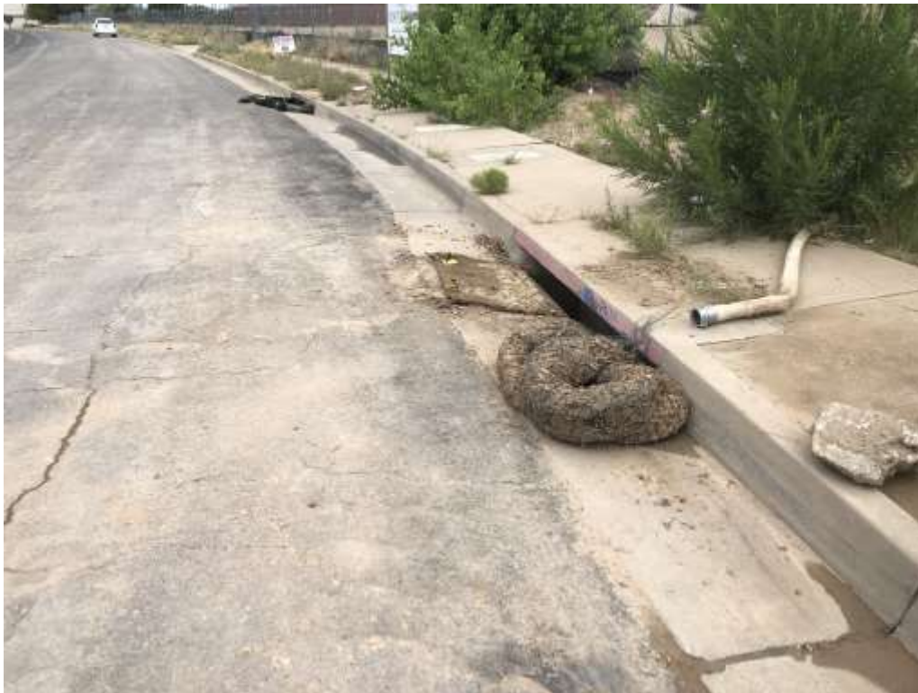
Clear Area of Sediment and Replace or Install new wattles
