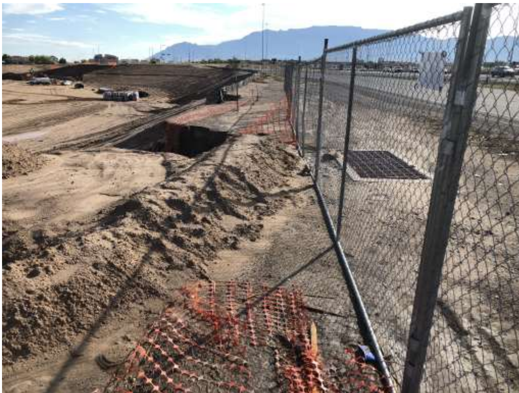
NMDOT Inlet Uncontrolled Run-On
