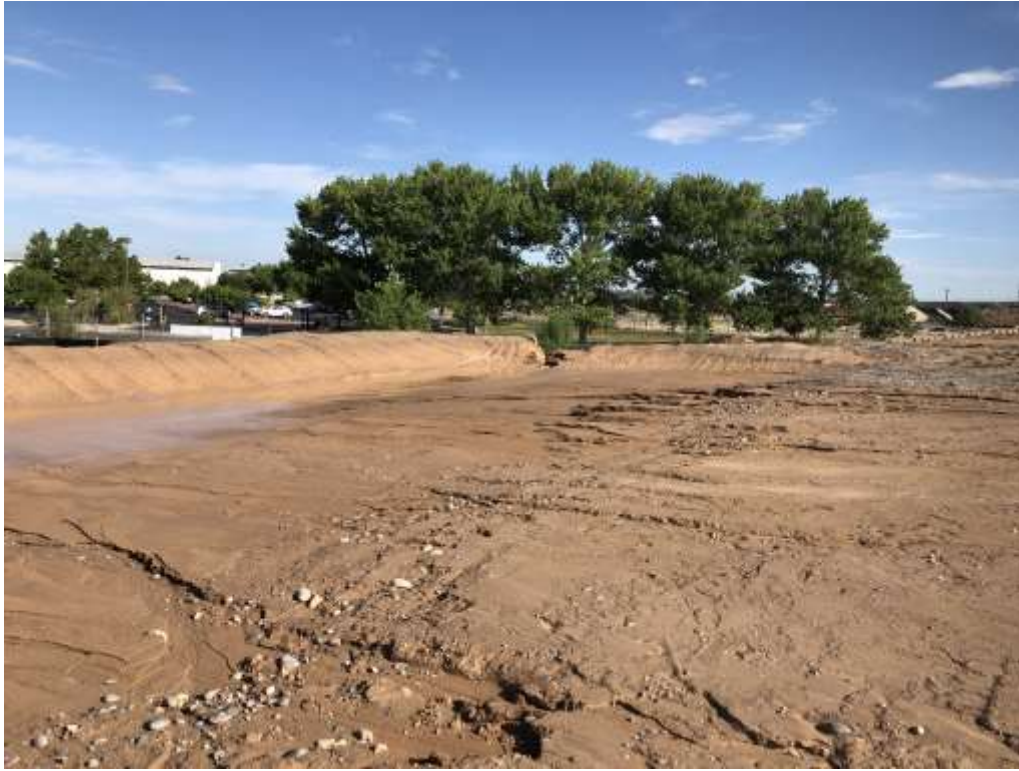
Sediment Trap Breach
