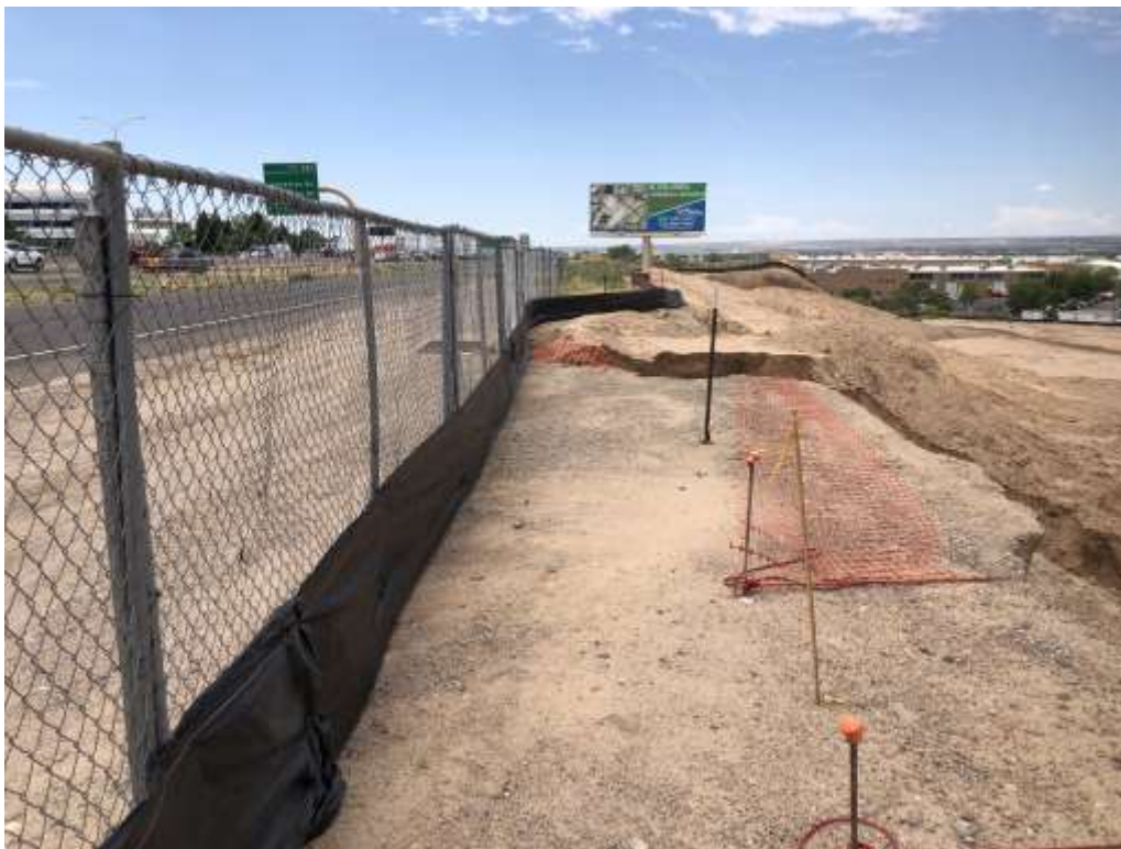
Berm or other diversion should be installed to direct flow towards inlet
