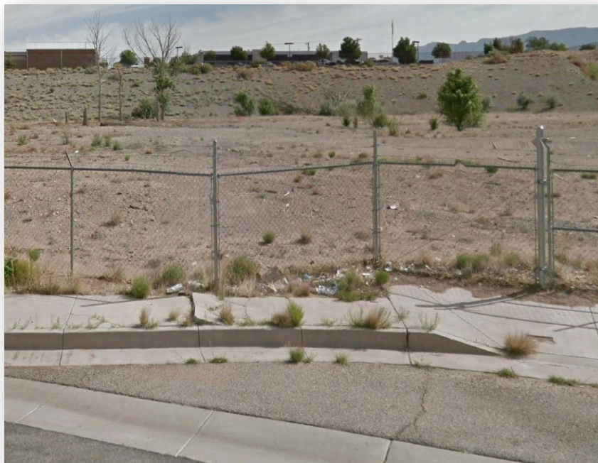
Sections Damaged Due to Expansion
