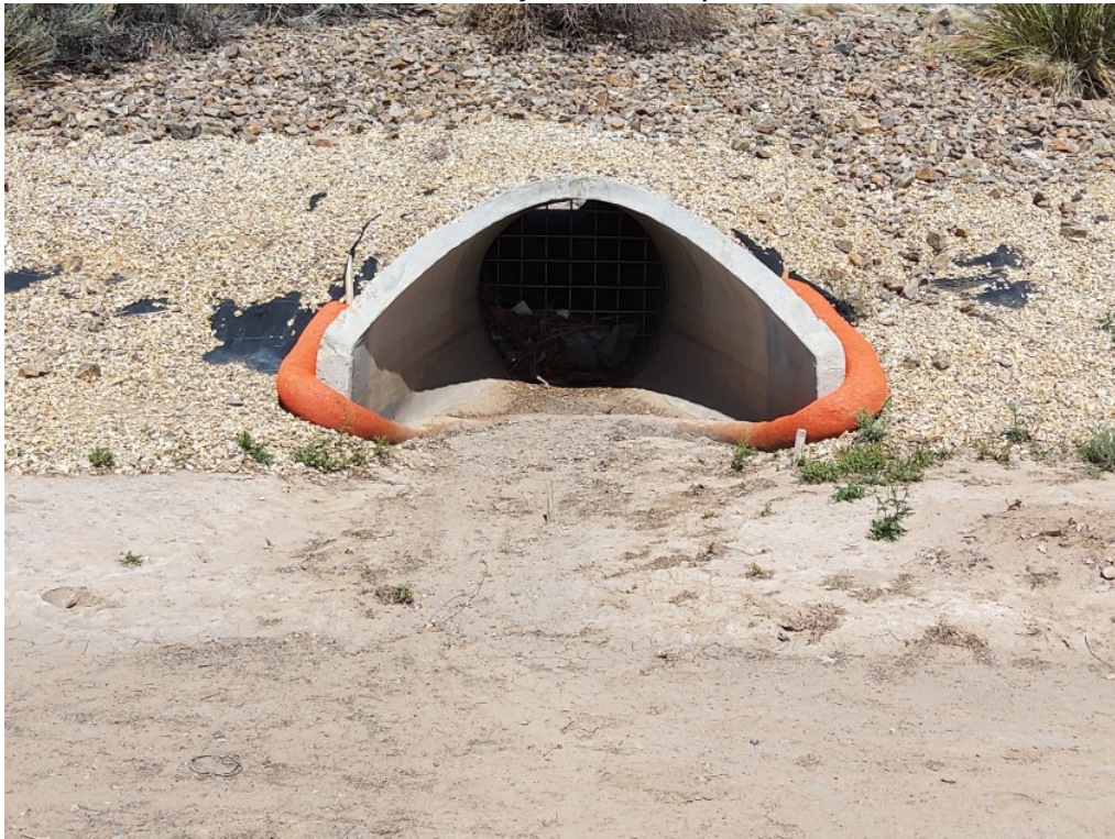
Site Walk Deficiency Photos - Inlet protection
