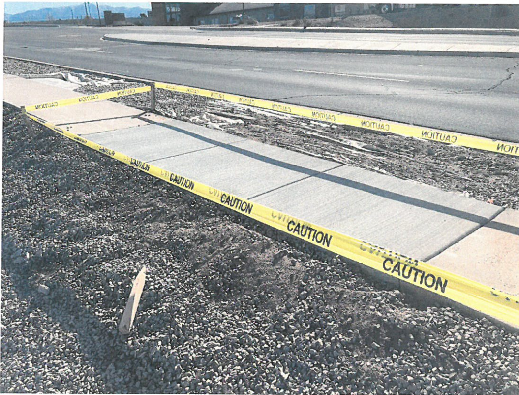
Sidewalk heaving has been replaced
