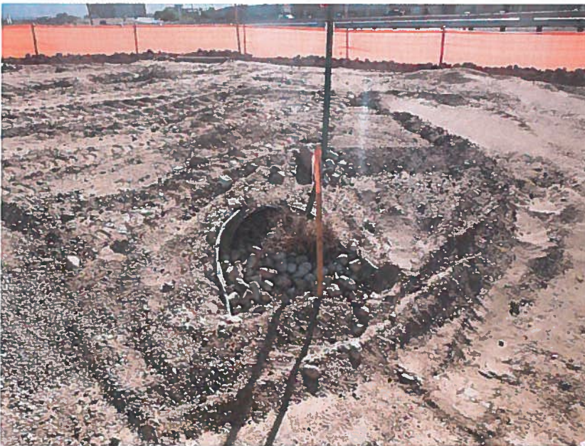
Northeast culvert that needs cobbles removed.
