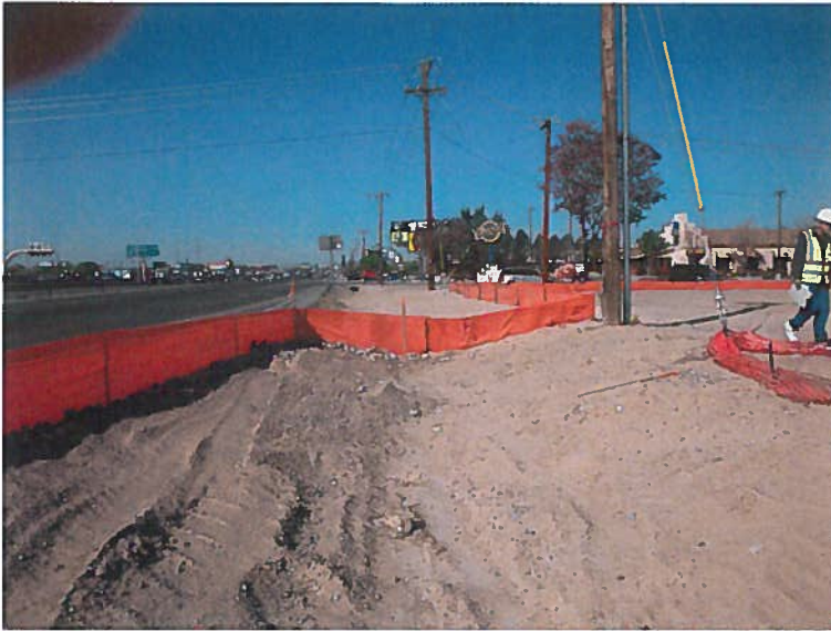
Silt fence at southeast corner to be removed and replaced with appropriate material
