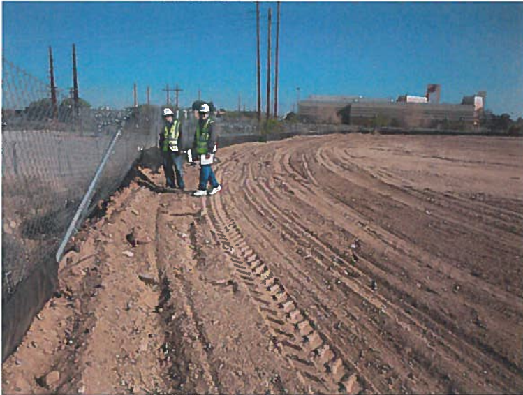
Southside of site that needs to be graded to sediment basin.
