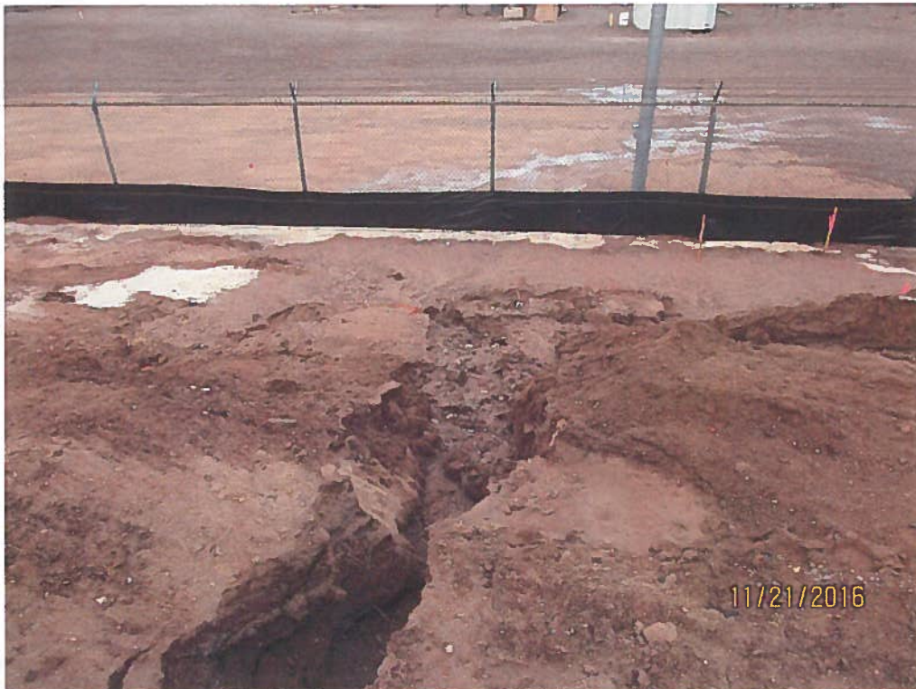
Arroyo draining into PNM substation. Area is also eroding.
