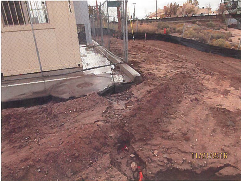
Location where drainage leaves the parking lot.
