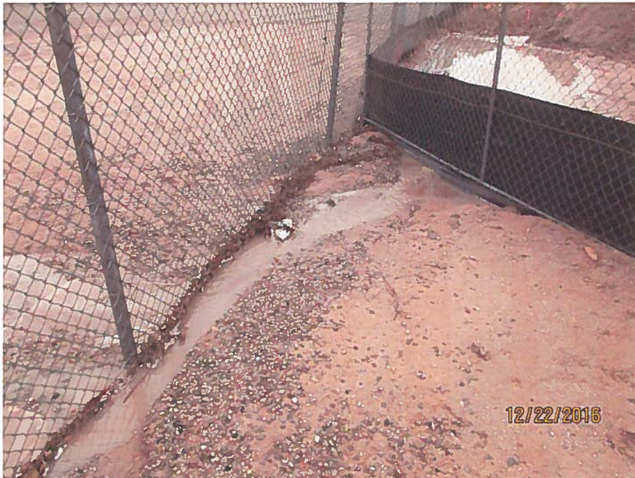
Drainage leaving site.
