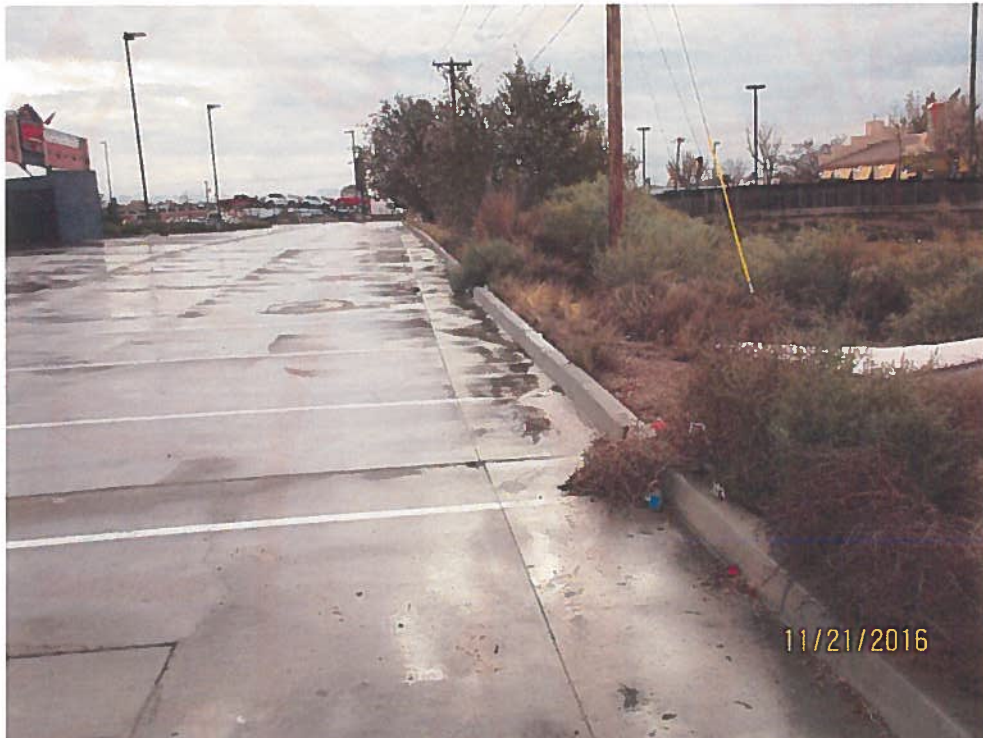
Portion of drainage basin draining to PNM substation.
