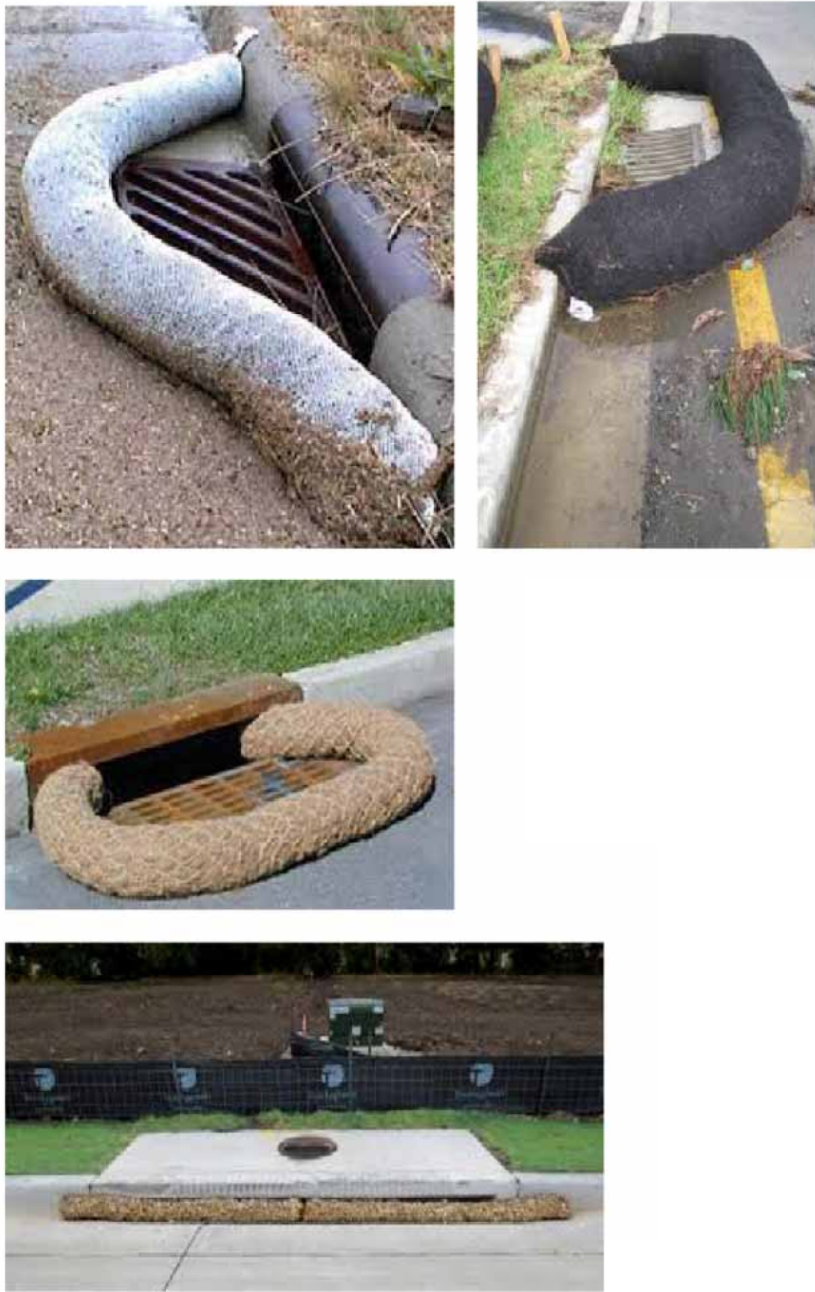
Curb Storm Inlet Protection with Wattles
