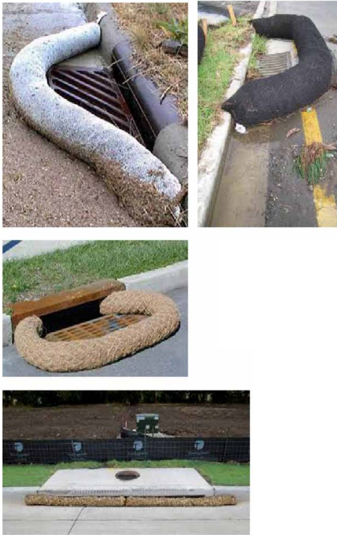
Curb Storm Inlet Protection with Wattles
