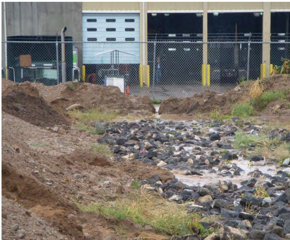
5: HAND EXCAVATED CONTROLLED RELEASE OUTLET
