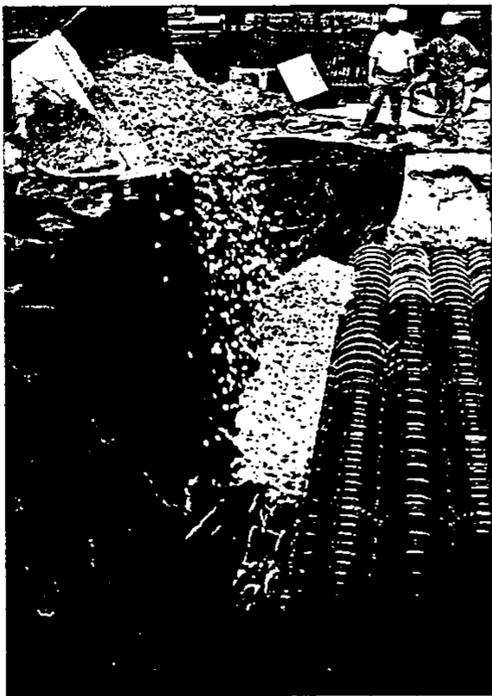
*Note: If the inletting system uses perforated pipe at the perimeter of the bed, rather than a header and manifold configuration, crushed stone must be placed in lifts with the top of the first lift at the planned elevation of the bottom of the feeder pipe.*
