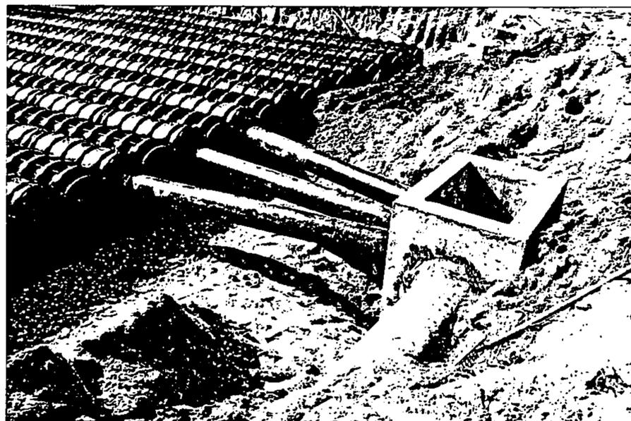
Run the distribution pipe to the chamber rows from the catch basin or other sedimentation structure.
