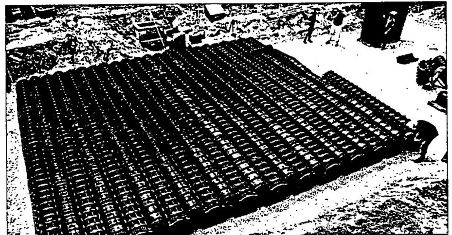
Each time you place a Maximizer chamber, the connecting two PowerArch bridges must be installed.
