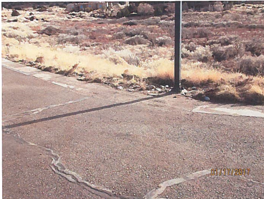
Dirt at vegetated area.
