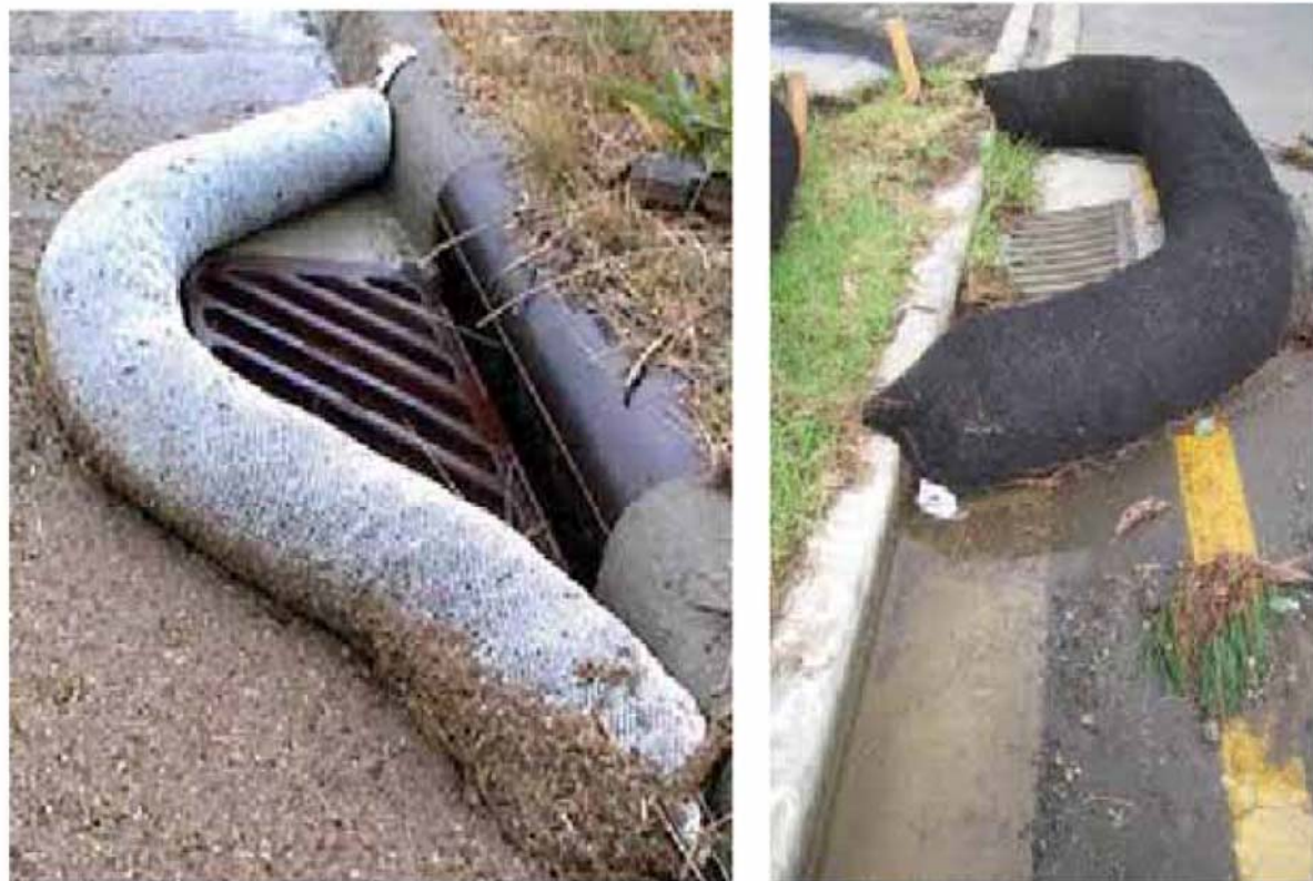
Curb Storm Inlet Protection with Wattles
