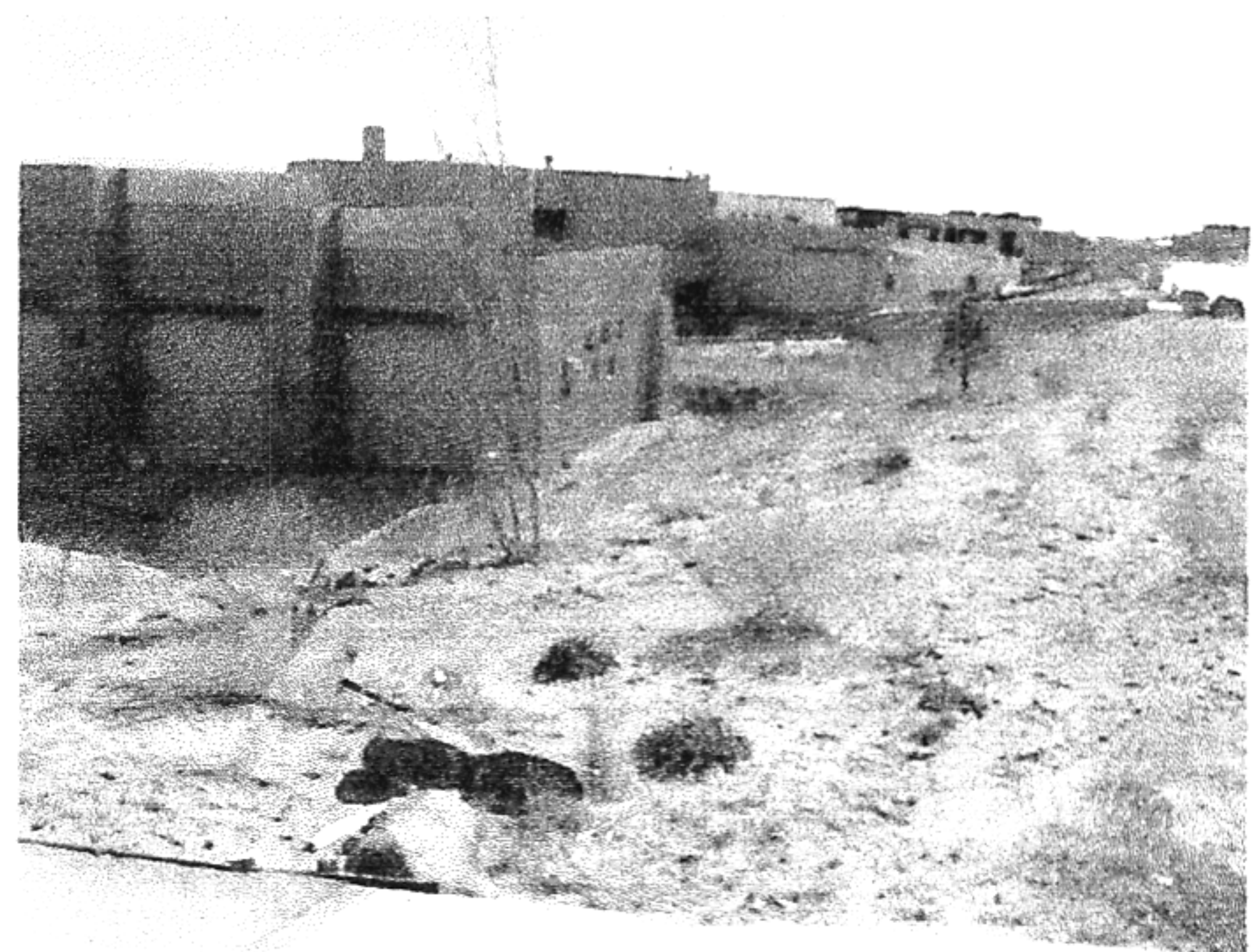
West Side looking South
