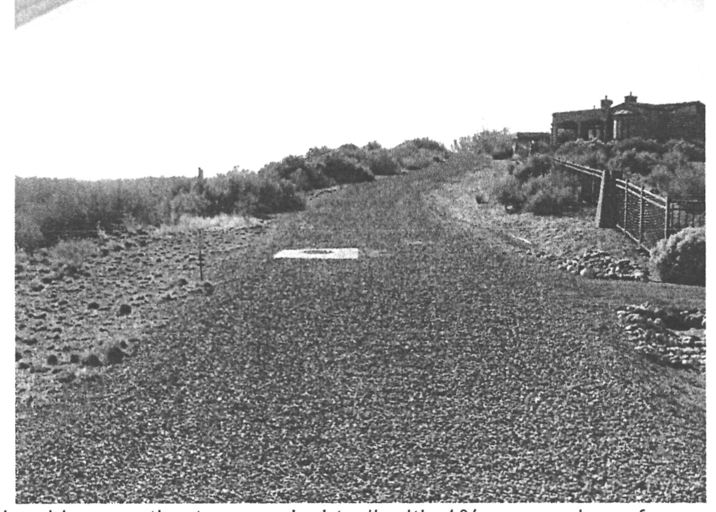
Photo 3 – Looking south at re-graded trail with 1% cross-slope from east to west
