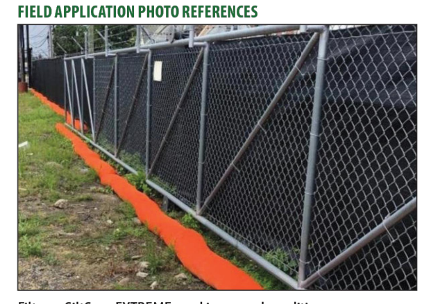
Filtrexx SiltSoxx EXTREME used in rugged conditions.
