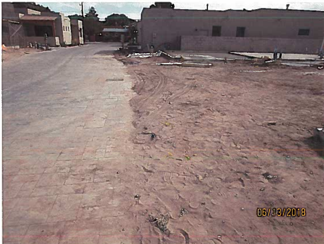
No sediment BMP and sediment in the street.
