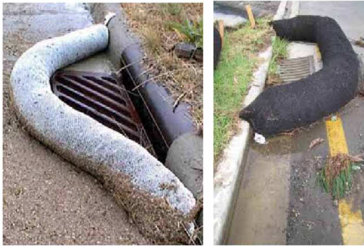
Curb Storm Inlet Protection with Wattles
