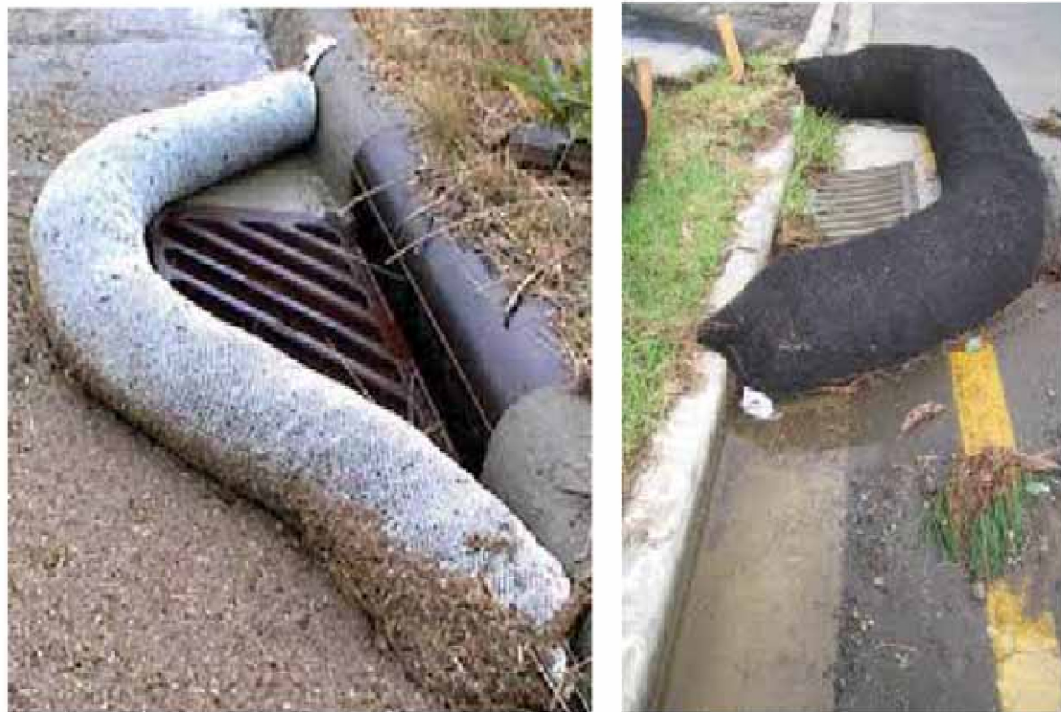
Curb Storm Inlet Protection with Wattles
