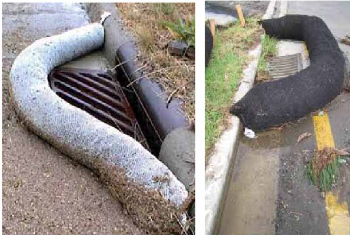
Curb Storm Inlet Protection with Wattles
