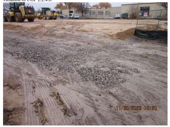
Inlet protection measures were missing. So they failed to remove sediment from this site prior to entering the storm drain inlets downstream from this site.
