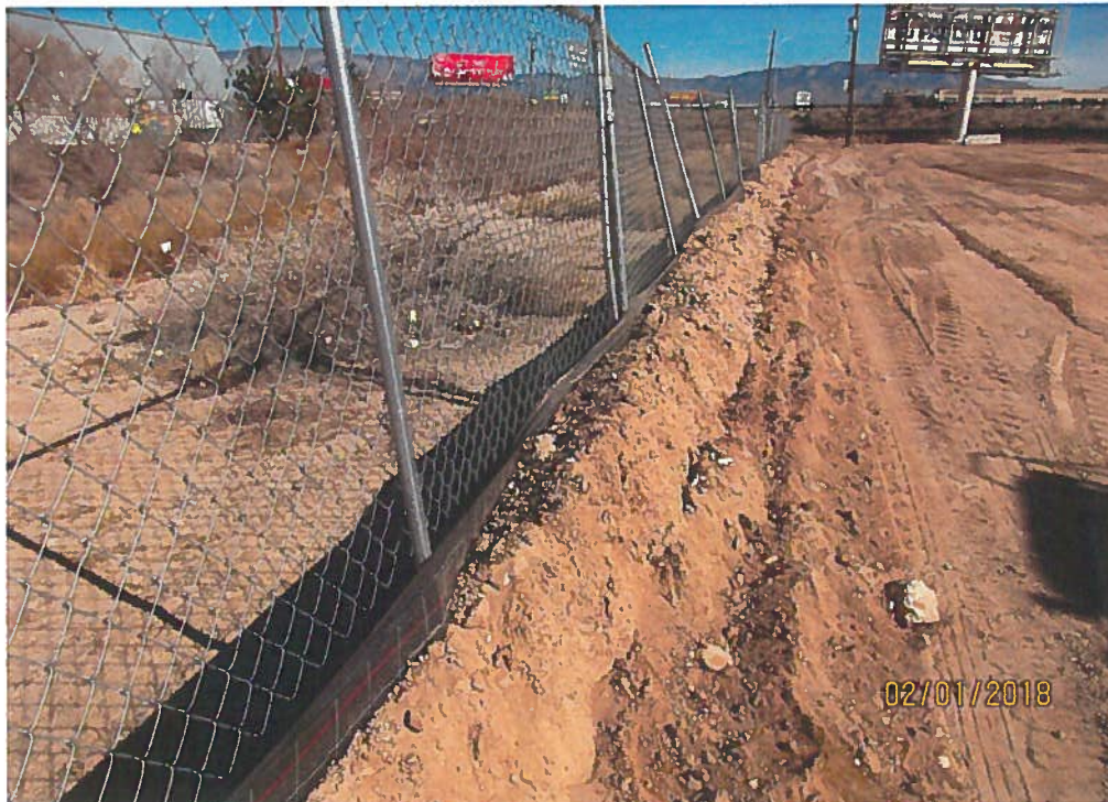
Grade too high against silt fence on north side of the site.
