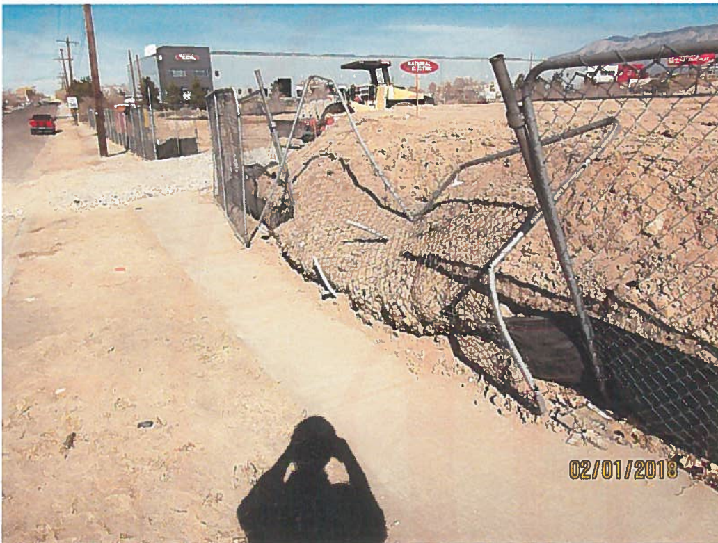
Too much dirt graded against silt fence caused a breach. Sediment on the sidewalk.
