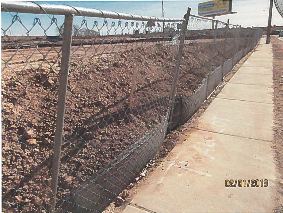
Grade too high against silt fence on west side of the site.
