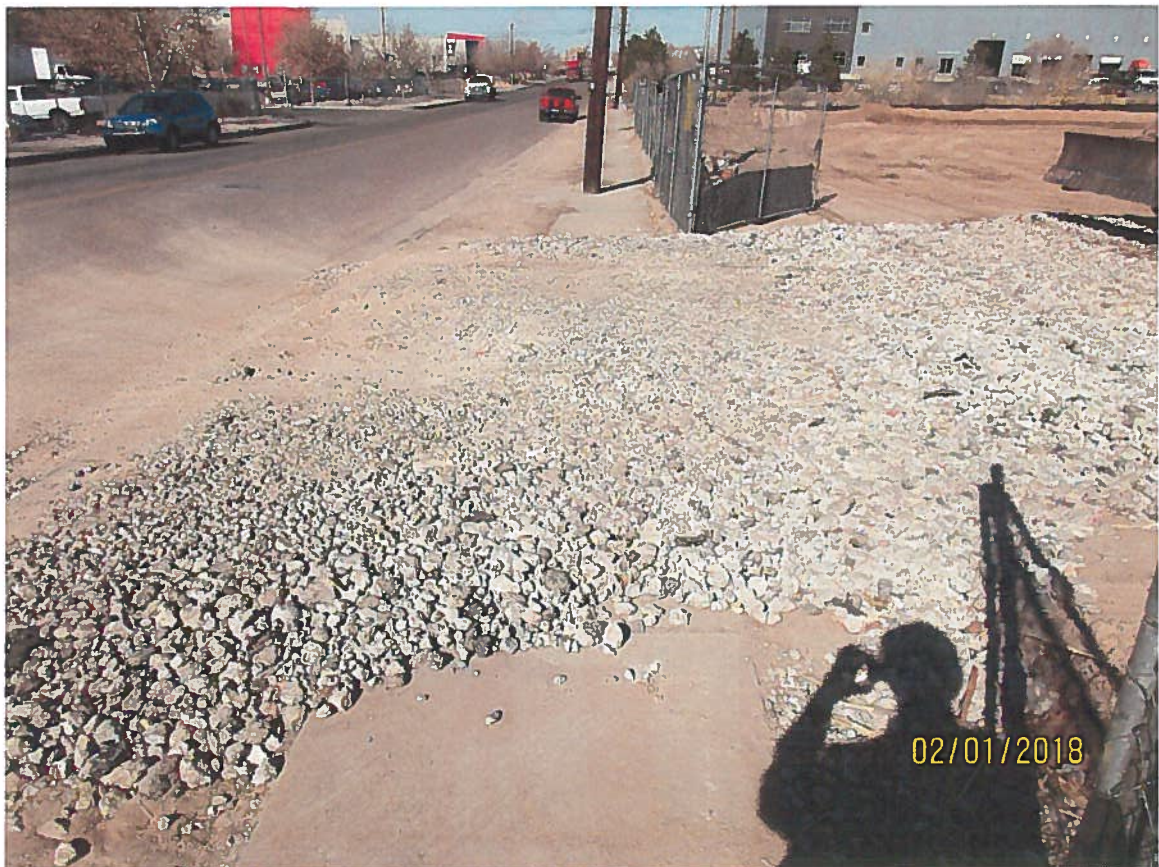
Track-out pad built over the sidewalk.
