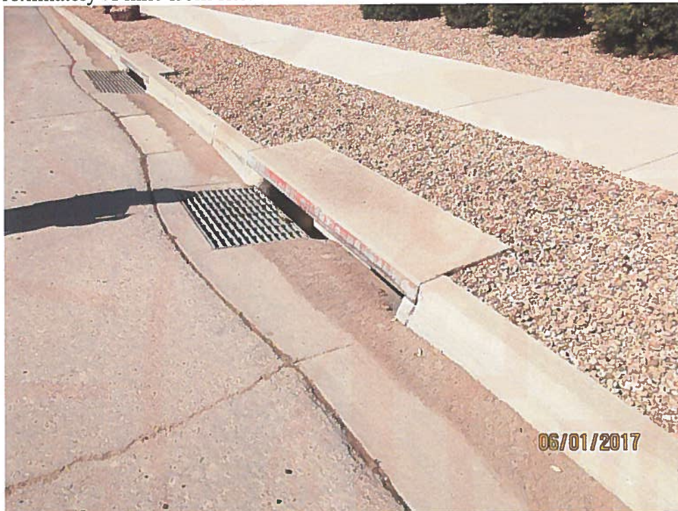
Inlet on Vassar Dr with sediment.
