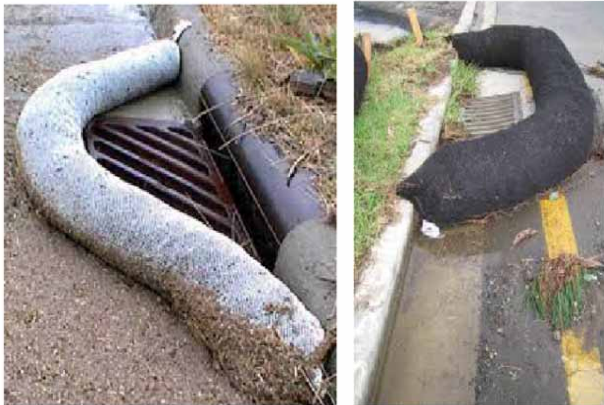
Curb Storm Inlet Protection with Wattles
