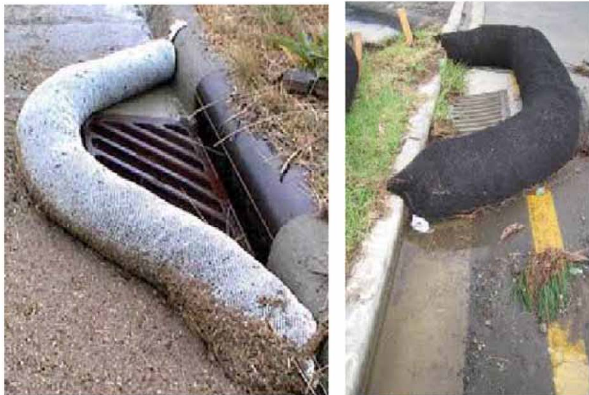
Curb Storm Inlet Protection with Wattles
