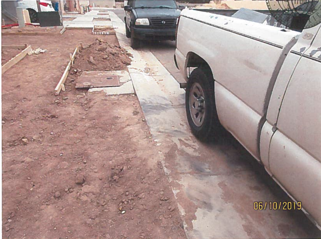
Sediment in street and gutter and no sediment BMP.
