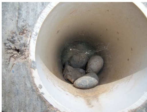
Figure 5: Weep Hole
