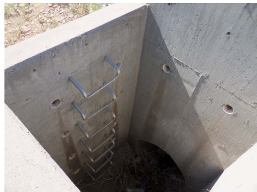
Figure 6: Pond Outlet Structure
