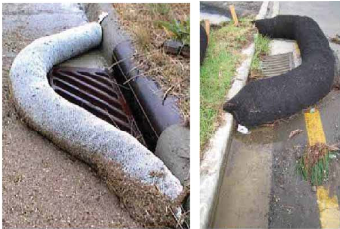
Curb Storm Inlet Protection with Wattles
