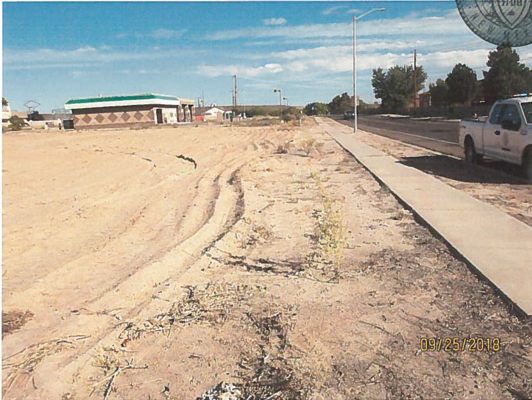
No sediment BMP east edge.
