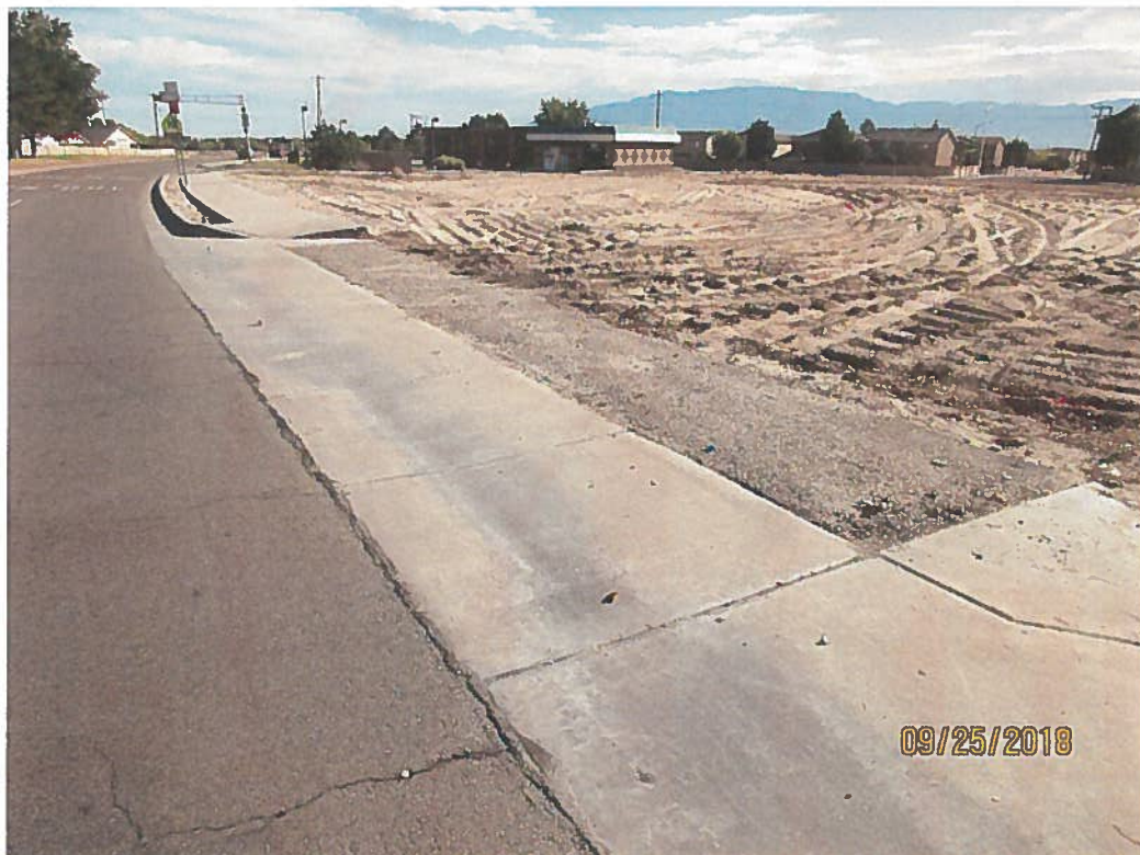
Site exit with no vehicle tracking control.
